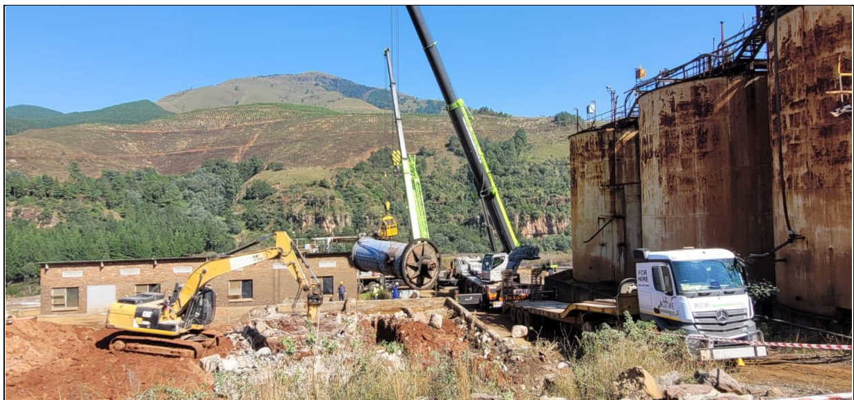
Figure 4: Breaking of old mill civis and loading of ball mill
