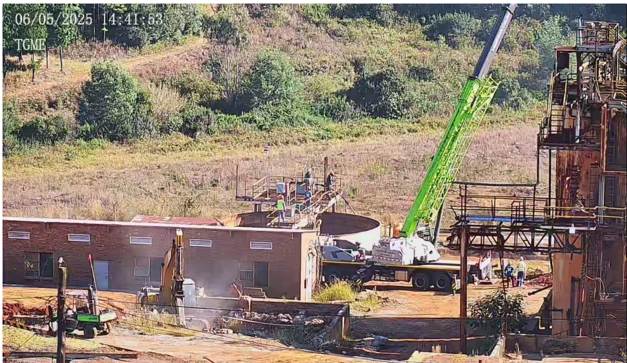
Figure 2: Removal of old mill civils and thickeners
