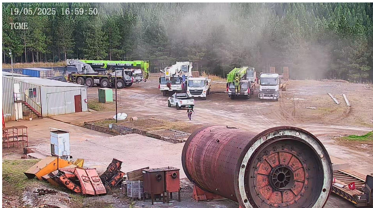
Figure 1: Mobile Cranes and Flatbed Trucks assisting in deconstructing the old plant.
