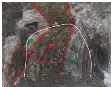
995 south ore drive (4.7mW x 4.5mH) with a face grade 3.8%
