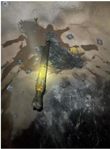
Shaft pilot-hole breakthrough at shaft bottom
