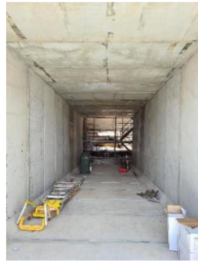
Cold air duct into shaft
