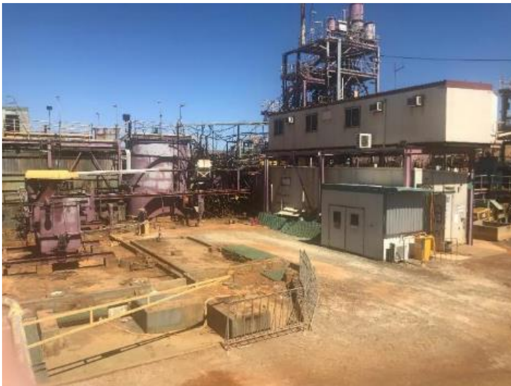
Cosmos Concentrator – Flotation cells and ISA mill removed
