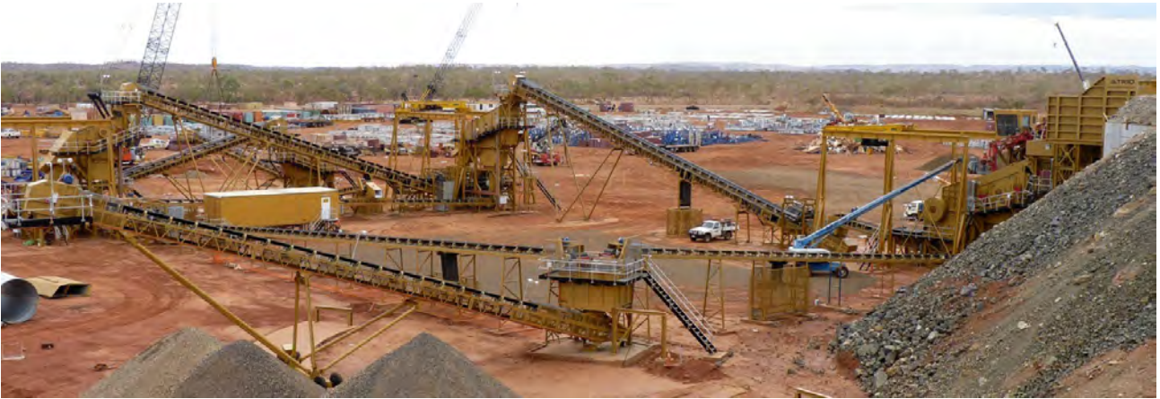
Figure 09: Crushing Circuit in foreground and numerous deliveries of steelwork and other componentry in the lay-down area in the background
