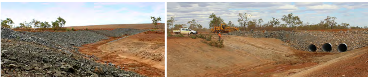
Figure 19: Armor rock surfacing on the MCD channel (left) and on culverts crossing the MCD channel (right)
