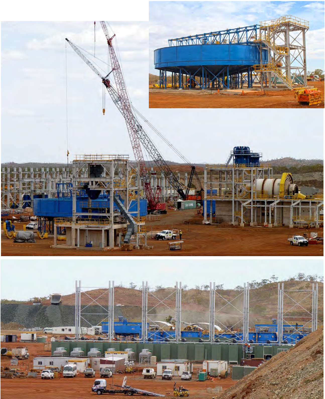
Figure 08: From top to bottom; Gravity Thickener (completed), Ball Mill, HPGR and Gravity Thickener and; Power Station
