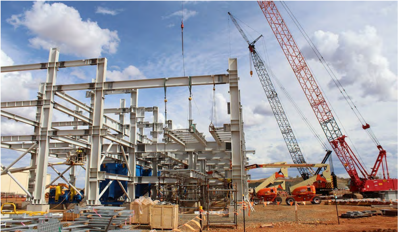
Figure 11: Structural framework being erected at the gravity jig building.
