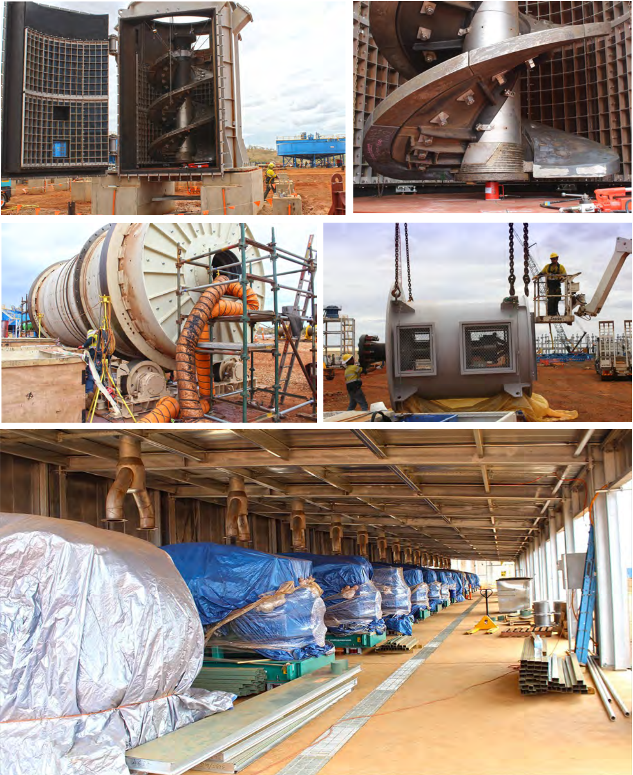
Figure 15: Tower Mills and assembly, De-agglomerator and gen-sets at the Power Station
