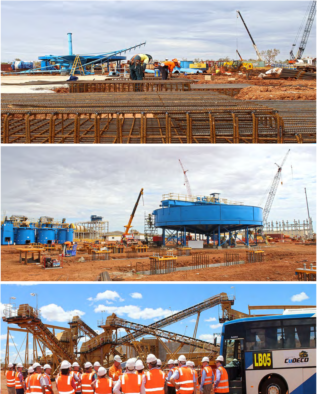
Figure 13: From top to bottom; Footing being constructed for the Flotation Cells; Concentrate Thickener and; shareholders inspecting the Crushing Circuit during the Company's 2013 AGM.
