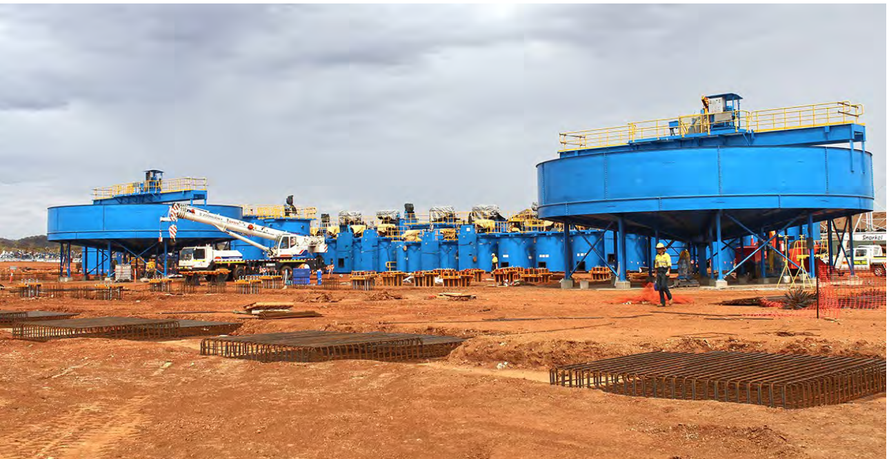
Figure 14: Top to bottom; Grinding Circuit and; Concentrate Thickeners and Flotation Cells
