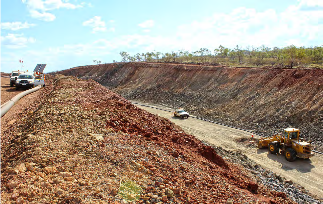
Figure 29: Solar powered water-flow monitor being installed ion the MCD channel.
