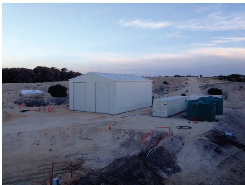
Onshore Garden Island showing (from left to right) power house, containerised desalination plant and water storage tanks
