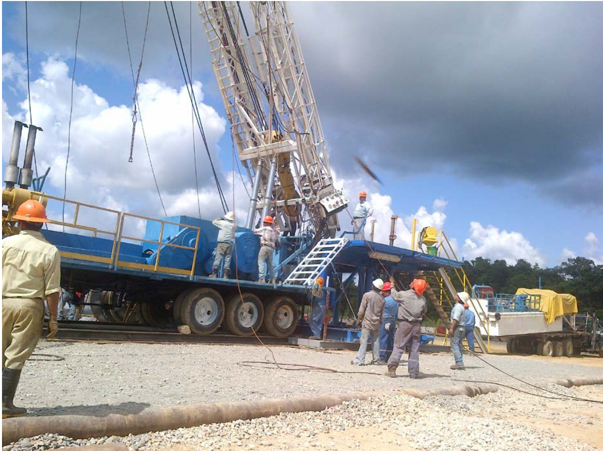
Rigging up mast on Atzam #5 location
