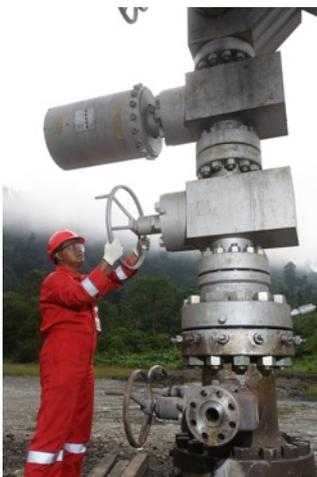
Figure 2 Pase A-2 wellhead
