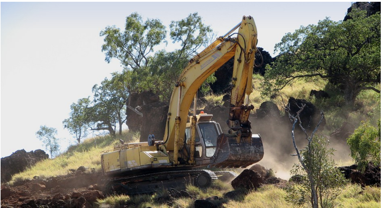
Figure 32: "Mozzie" clearing pads in difficult terrain at Wilgar. Limited access has hindered the exploration effort at Wilgar somewhat, with steep topography and rocky conditions severely limiting options for drill hole locations. A series of drill-pads are currently being cleared, to facilitate drilling from previously inaccessible locations
