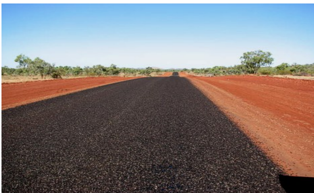
Figure 37: First of several bitumen layers to be applied
