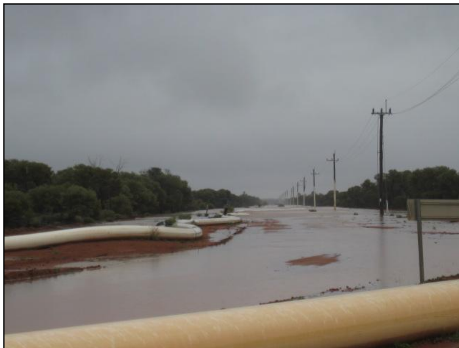
Pipeline at bore field shifted significantly from foundations by floodwaters
