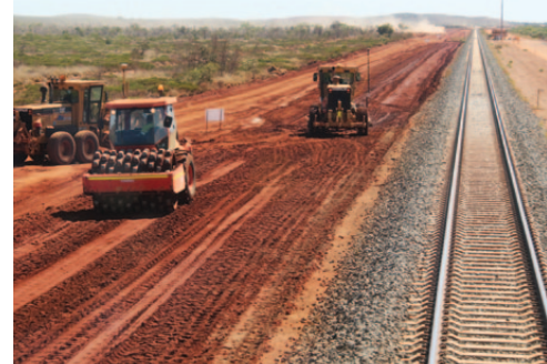
Top and below: Rail earthworks for mainline duplication
