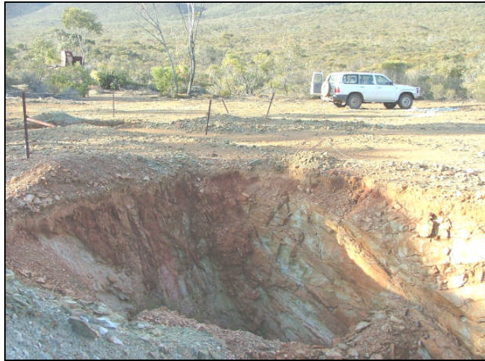
Figure 3: Looking North - Mt Desmond shaft in background, crown pillar mineralisation exposed in old working in foreground.
