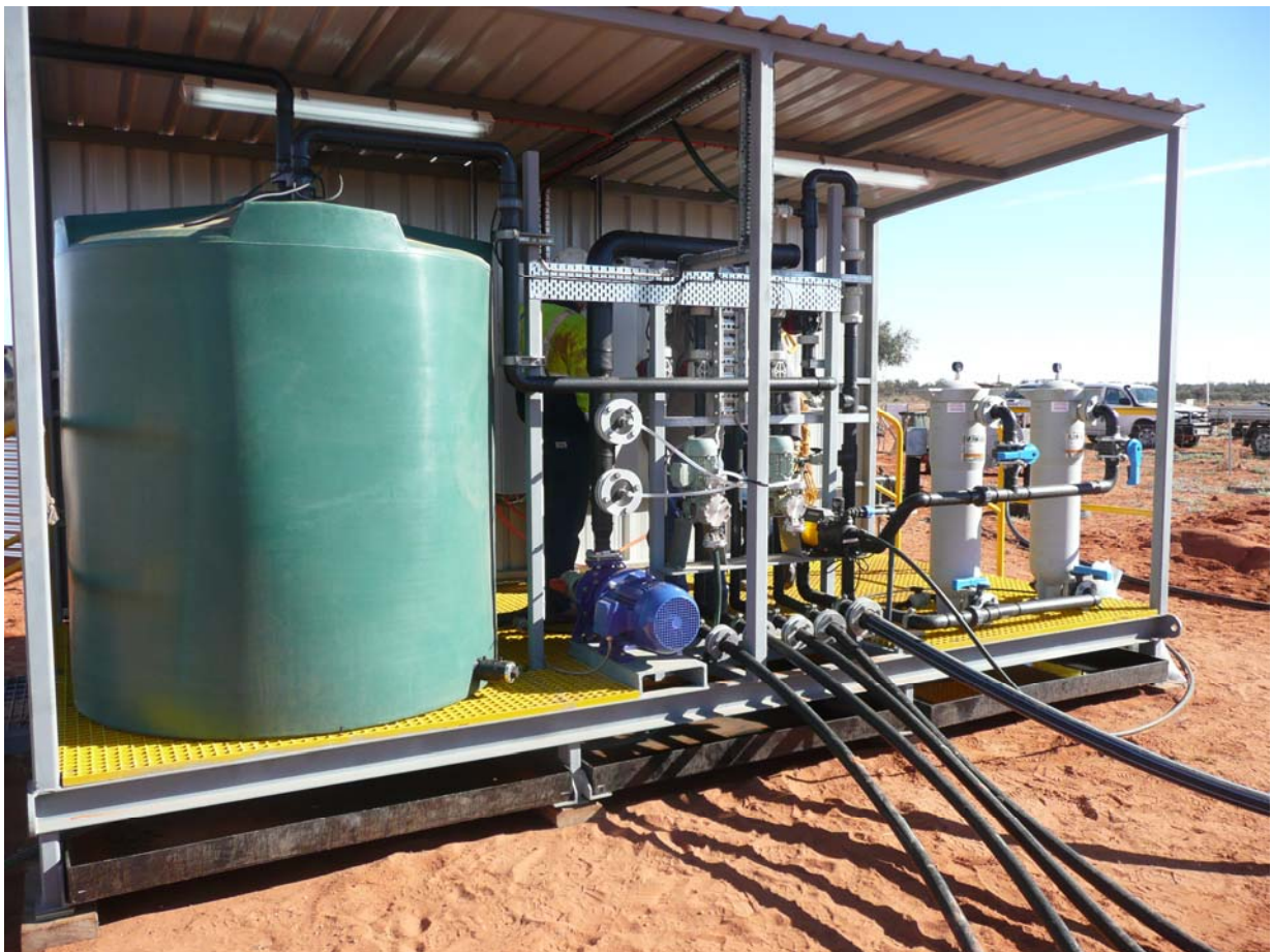
Figure 2 : Well house unit in operation on site
