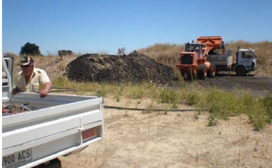
REMOVING OVERBURDEN TO PREPARE THE DIRECTIONAL DRILL SITE PAD
