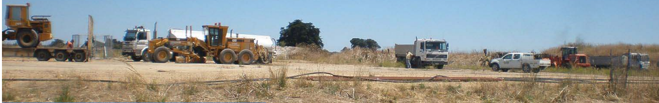
REMOVING OVERBURDEN TO PREPARE THE DIRECTIONAL DRILL SITE PAD
