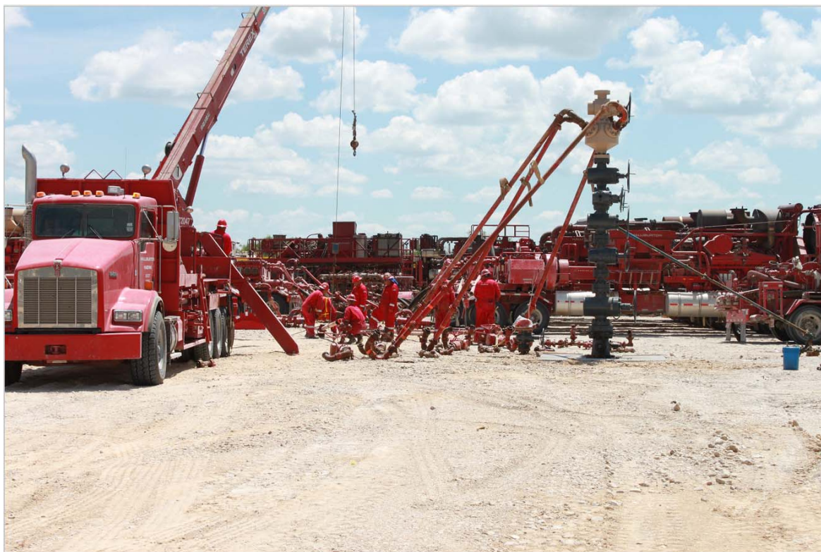
Halliburton personnel rigging up fracture stimulation flowlines on the Frances Dilworth No. 4H.
