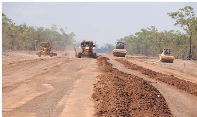
Haul road pavement construction
