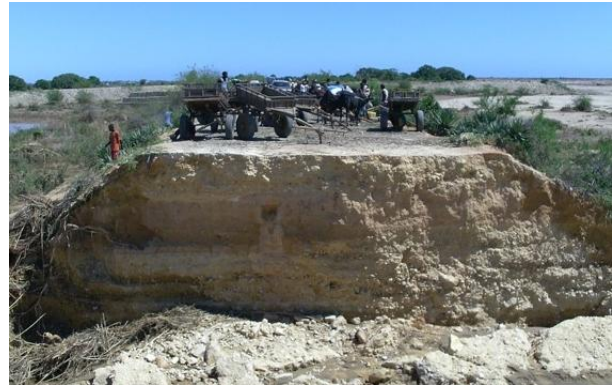
Fiheranana Bridge Access Washed Away
