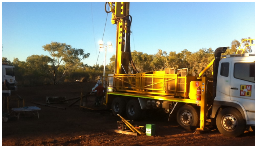
Figure 1: AMWD drilling completing Diamond Drill hole LBD4
