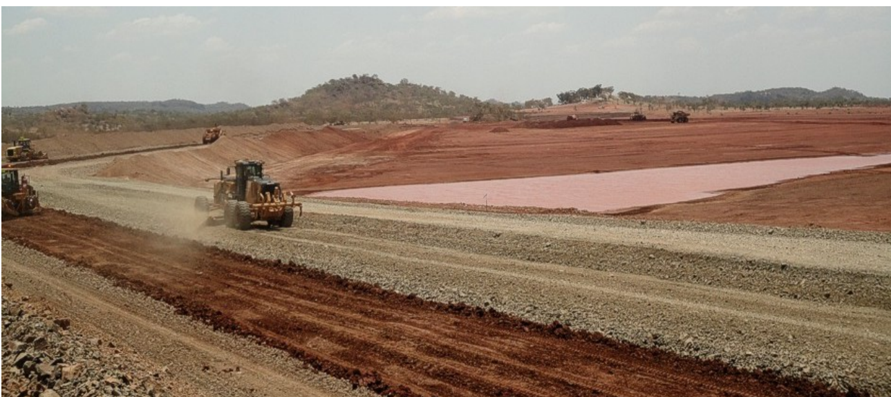
Figure 25: WSF Dam wall being build up around the iron-rich clays, easily distinguished from the light coloured (Corella Formation) rocks.
