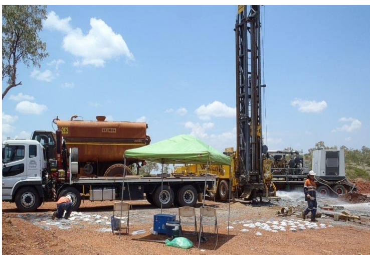
Figure 53: Pit-dewatering borehole drilling at Rocklands South towards the end of 2012. Significant water flow can be seen being ejected from the return pipe and samples for geological logging and assay (taken each 1m) are in the foreground - all holes intersected high-grade mineralisation
