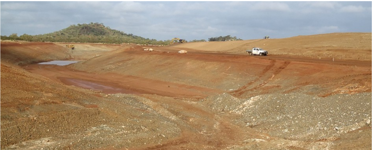
Figure 27: Morris Creek Diversion Channel (left) and Water Storage Facility dam wall (right) during construction.
