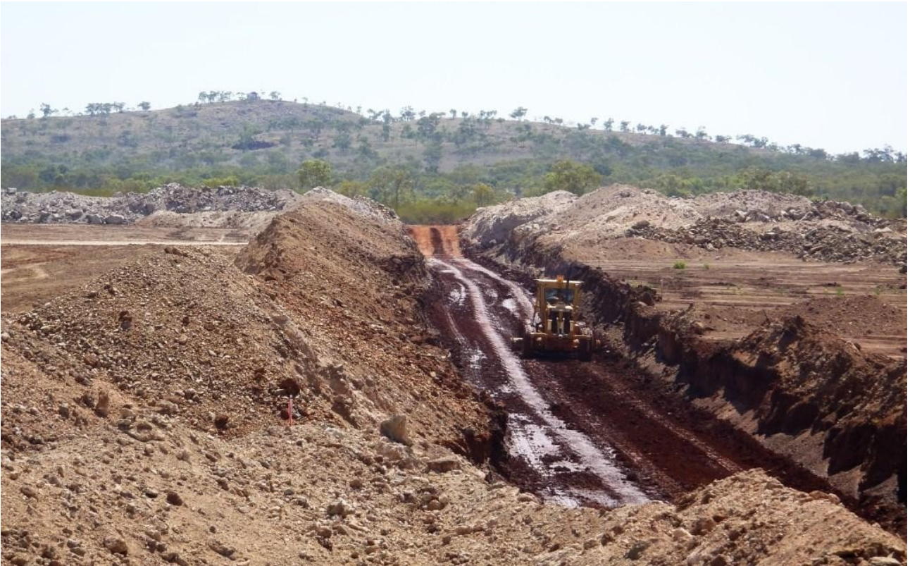
Figure 32: Water Storage Facility (WSF) key-way construction. Located beneath the WSF dam wall, the key-way is back-filled with water impervious clays that will continue to be built up as the dam wall sides are constructed, resulting in a water-impervious inner core.
