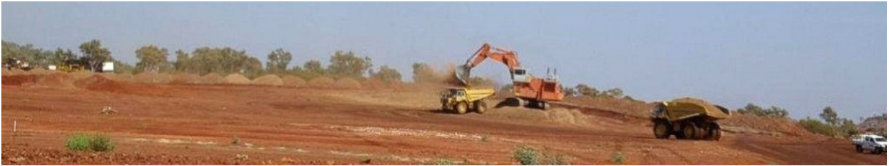
Figure 21: Free-dig material being removed from the northern end of the Las Minerale Pit area to be used for infrastructure earthworks such as the Water Storage Facility dam walls and Morris Creek Diversion Channel embankments. Some of the material is also being positioned around the lip of the surveyed pit outline, and will eventually be shaped into safety berms (barriers at the edge of the pit) once mining commences.
