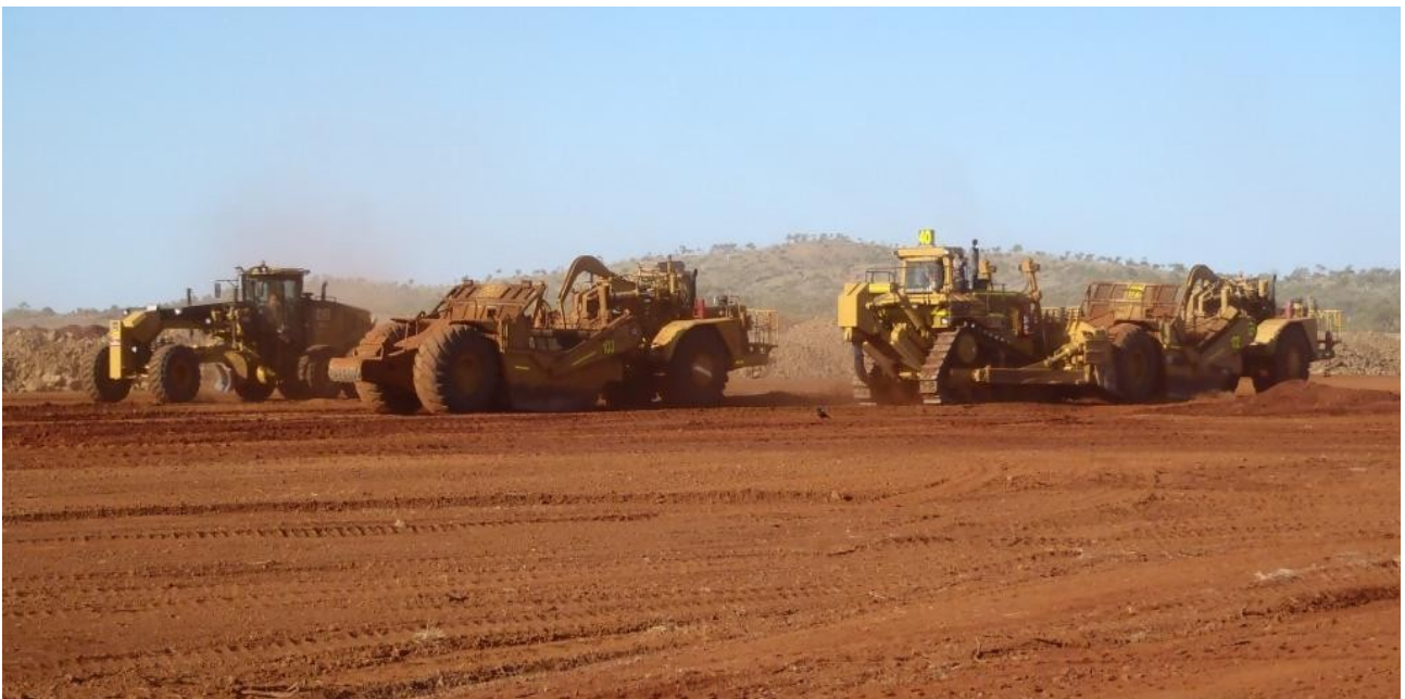
Figure 31: Pre-strip clearing of organic material and topsoil from the Process Plant area
