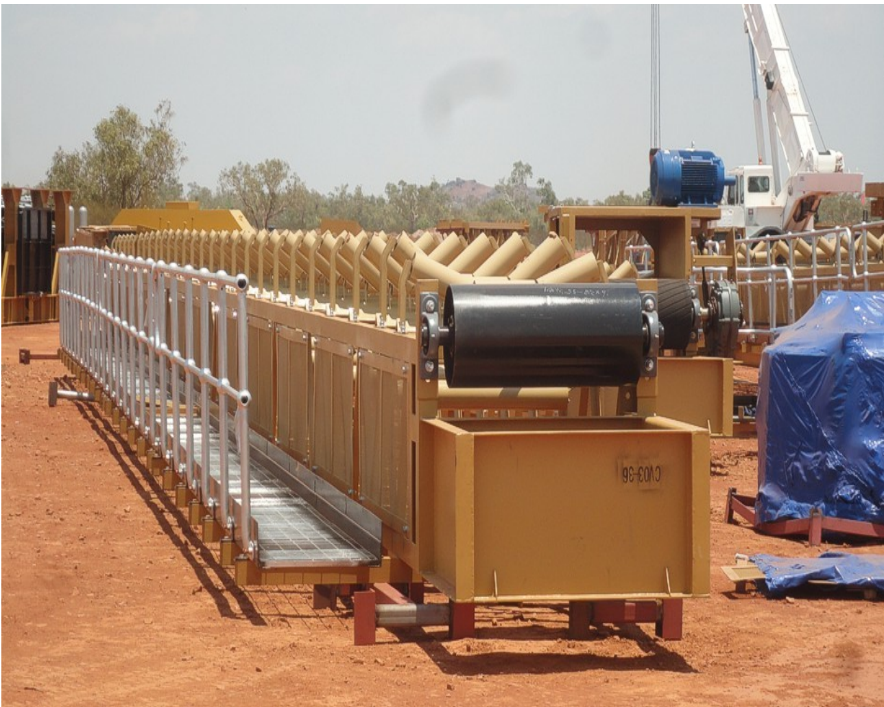
Figure 39: Various components of the plant have started arriving at site and will continue to be delivered over the coming months. Pictured is a roller conveyor...one of many that will eventually move product from one area of the plant to another.
