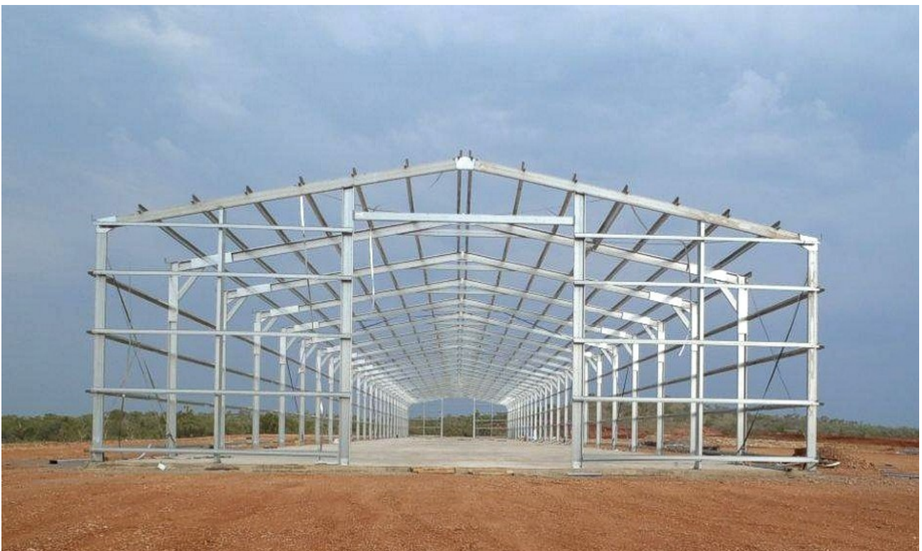
Figure 50: Process Plant Stores Area during construction
