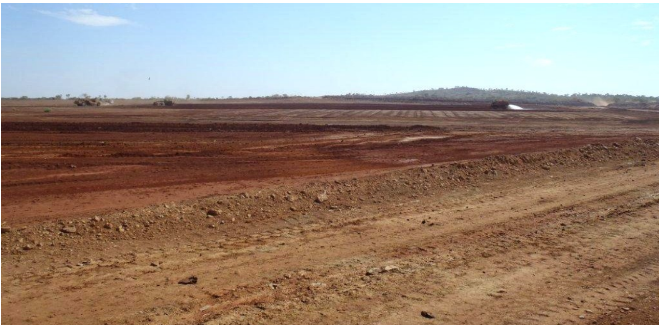
Figure 35: Water Storage Facility (WSF) - strip-back, levelling and clay distribution all but complete.
