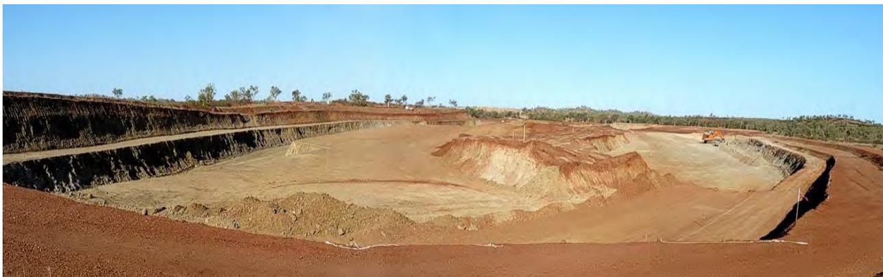
*Figure 12: North-west end of Las Minerale Pit (looking south-east), showing ore-zones left in centre of pit and waste areas either side being removed for use in various infrastructure requirements.*
