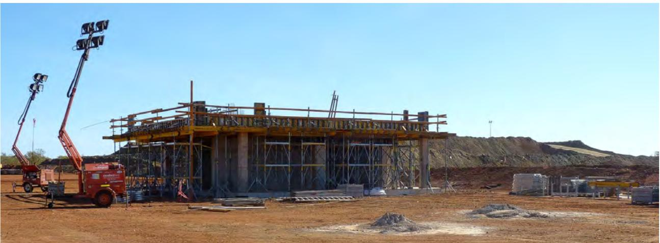
Figure 26: Ball Mill foundations with Crushing Circuit in Background (top image) and HPGR foundation with ROM Pad gradually being built up to the required level in Background (above image)
