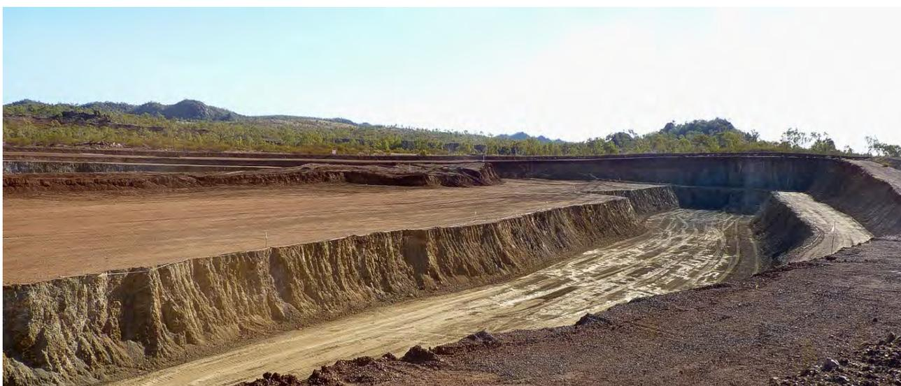
*Figure 13: North-west end of Las Minerale Pit, showing ore-zones left in centre of pit and waste areas either side being removed for use in various infrastructure requirements.*
