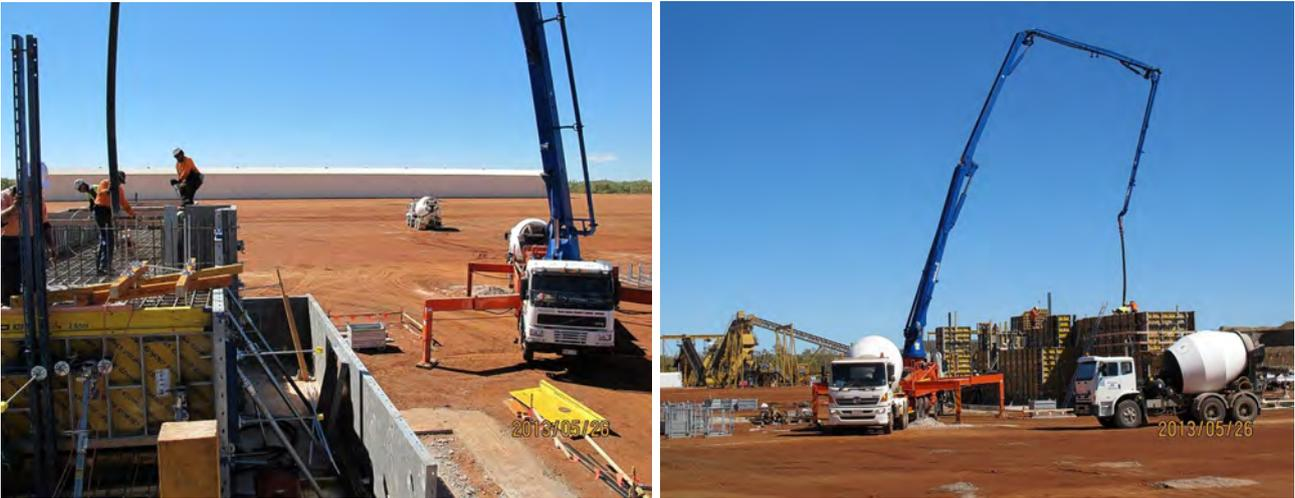
Figure 24: Massive concrete foundations for the Ball Mill being poured in stages, typically at night to avoid the heat of the day and premature curing, but recent mild weather has meant daytime concrete pours have been possible.
