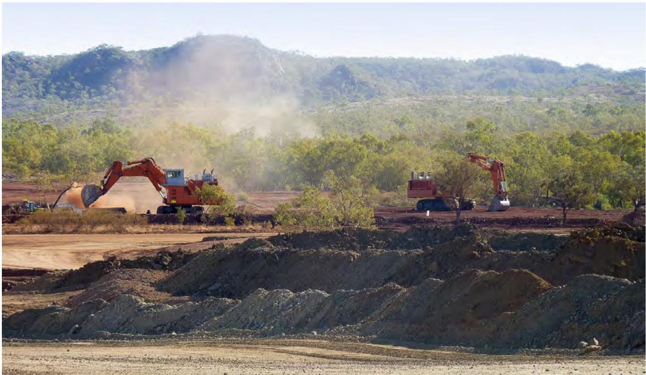
Figure 35: View from the ROM Pad looking towards the eastern end of the Las Minerale Pit, which has just started and will eventually be excavated to the same level (RL215) as the north-west end.
