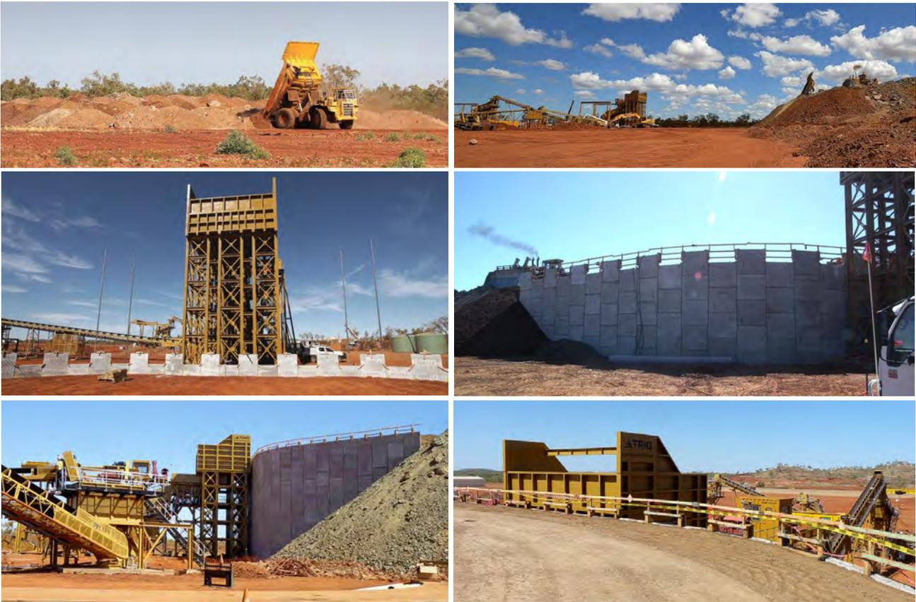
*Figure 43: Top to bottom; first loads of waste form the base of the ROM pad, which builds as more waste is added and the ROM grows towards the Crushing Circuit feed bin and construction of the ROM retaining wall commences and reaches final compacted height in the bottom-right image. The crushing circuit is undergoing final audit and minor completion tasks and commissioning is expected to take place as soon as the Run of Mine (ROM) pad has been completed and certified ready for use.*
