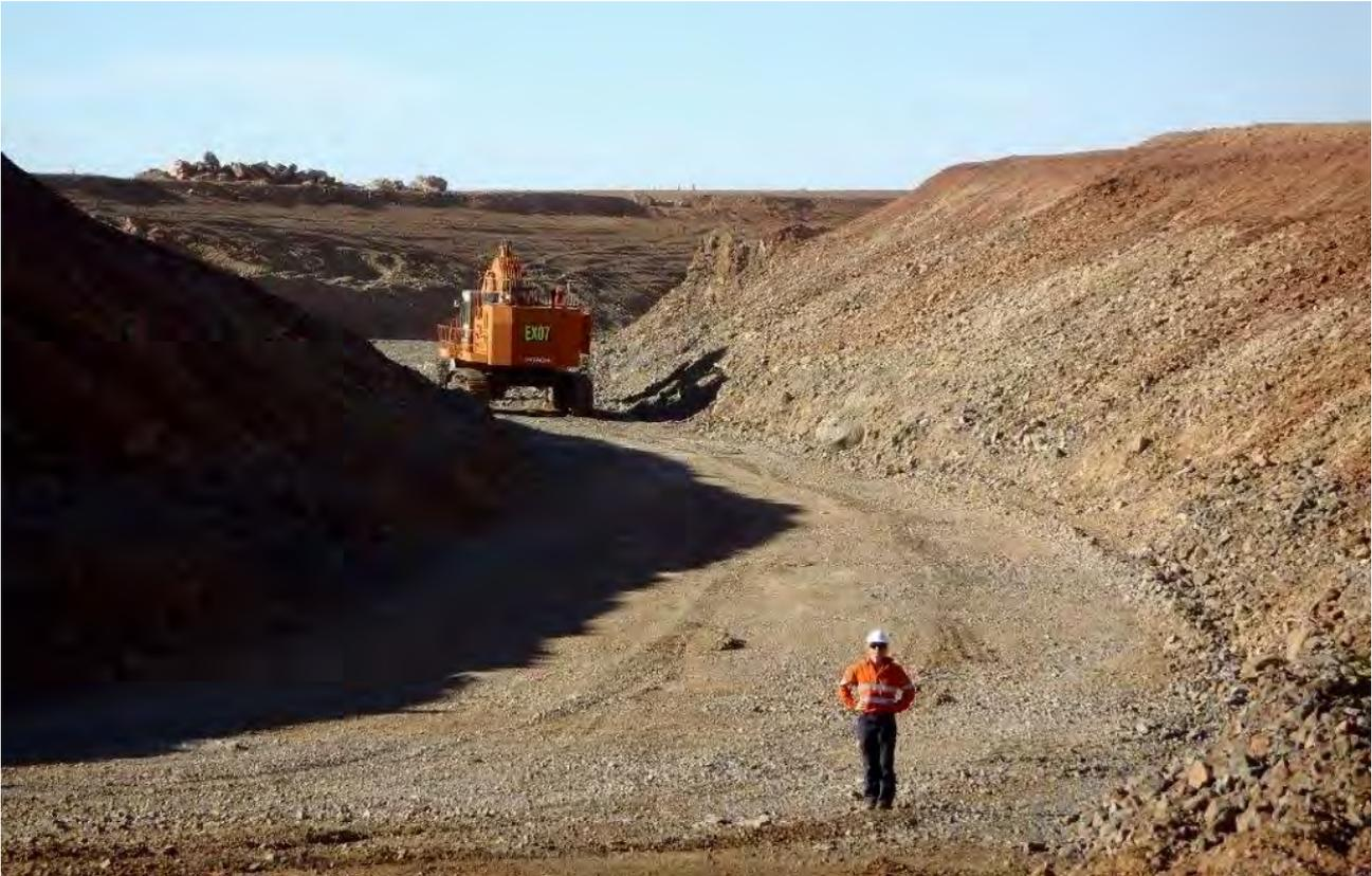
*Figure 31: Morris Creek Diversion Channel nearing completion, capable of withstanding a 1-in-100-year flood event. Interestingly, this actually transpired at Rocklands a few years ago, in spite of which Morris Creek (which the diversion channel is designed to re-direct) flowed running water for just one day and reached a flood height of approximately 1m.*
