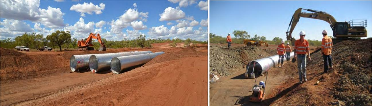
Figure 34: numerous culverts and water crossings are constructed as part of constructing the road infrastructure.
