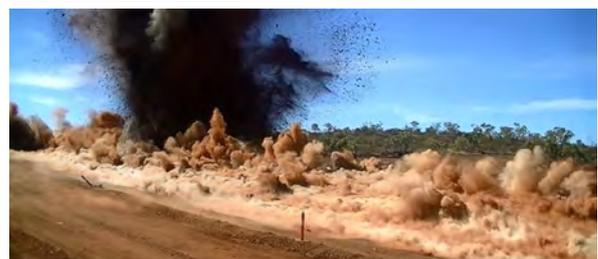
Figure 33 (top to bottom); Drill and blast - last shot to be fired at the Morris Creek Diversion Channel
