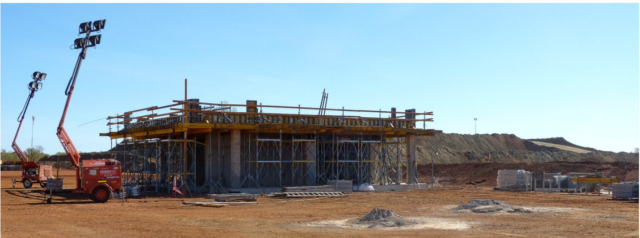
Figure 9: Ball Mill foundations with Crushing Circuit in Background (top image) and HPGR foundation with ROM Pad gradually being built up to the required level in Background (above image)
