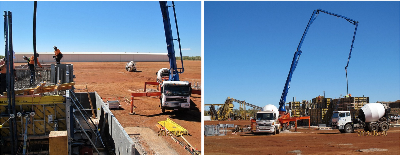
Figure 7: Massive concrete foundations for the Ball Mill being poured in stages, typically at night to avoid the heat of the day and premature curing, but recent mild weather has meant daytime concrete pours have been possible.
