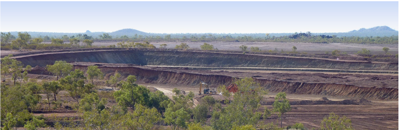
Figure 18: Las Minerale Pit (looking north-west from Telstra Hill); benches on the side of the pit taking shape as the entire LM Pit area is excavated to a single level (RL215) (top image) and; ore-zones left in centre of the pit at the north-west and of the Las Minerale Pit (above image)
