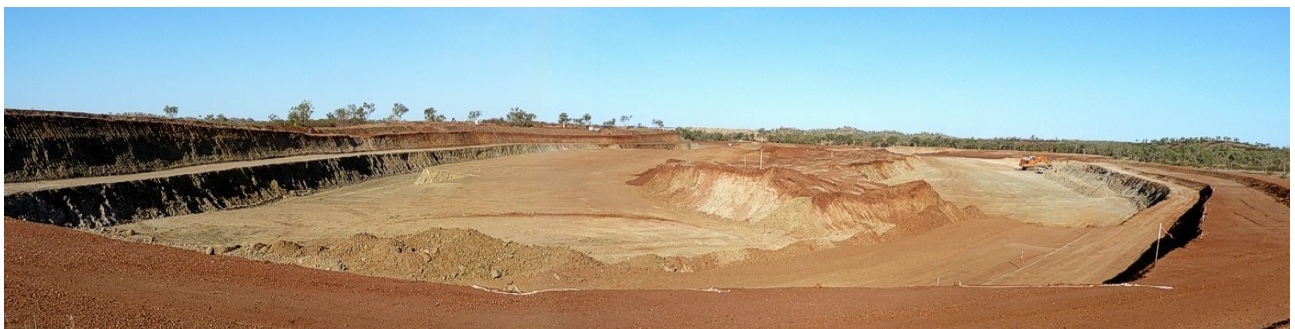
Figure 12: North-west end of Las Minerale Pit (looking south-east), showing ore-zones left in centre of pit and waste areas either side being removed for use in various infrastructure requirements.
