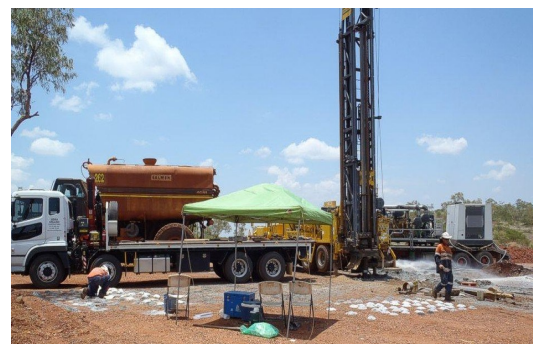
Figure 3: Pit-dewatering borehole drilling at Rocklands South towards the end of 2012. Significant water flow can be seen being ejected from the return pipe and samples for geological logging and assay (taken each 1m) are in the foreground - all holes intersected high-grade mineralisation.
