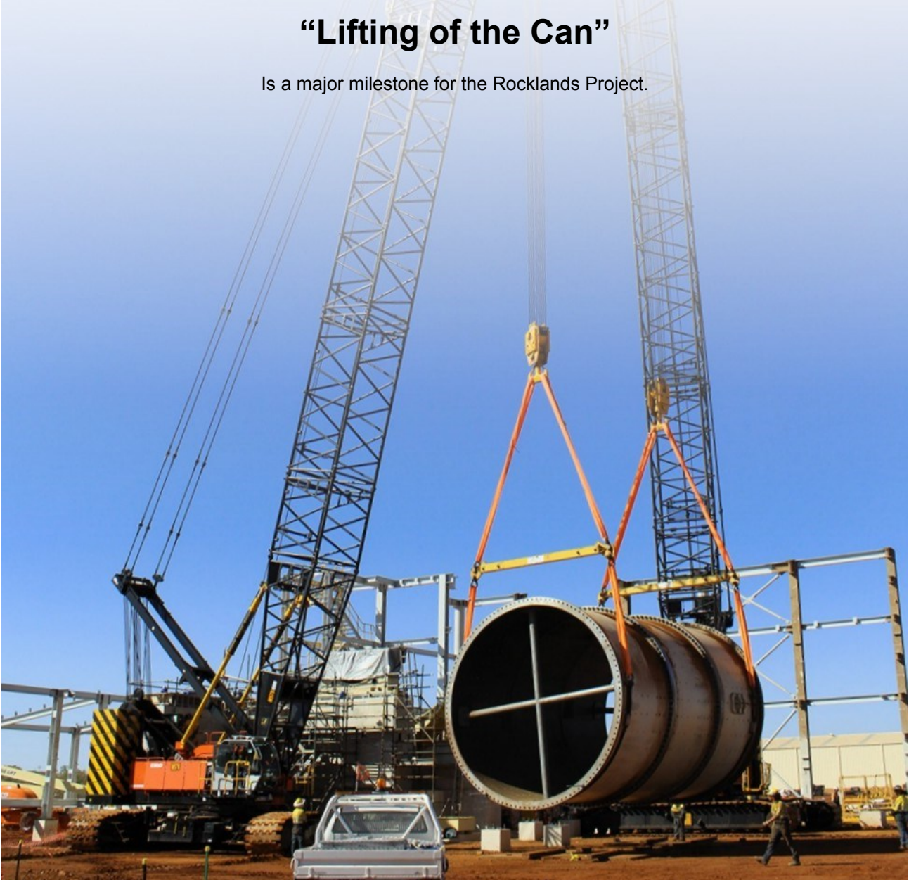
Figure 1: Two 250 tonne Waltz heavy-lift cranes begin lifting the Ball Mill into place.
