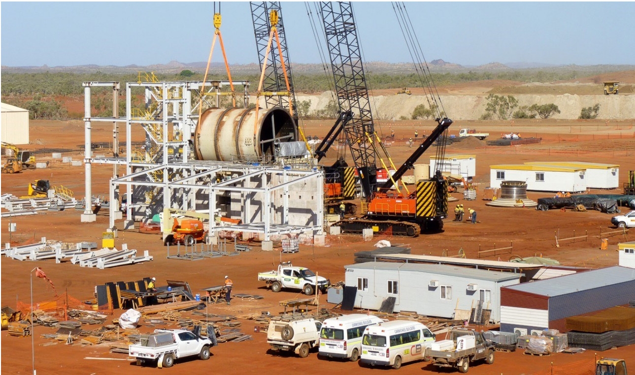
Figure 5: View from the ROM Pad of Ball Mill drum being installed - the ends can be seen to the right of the cranes.
