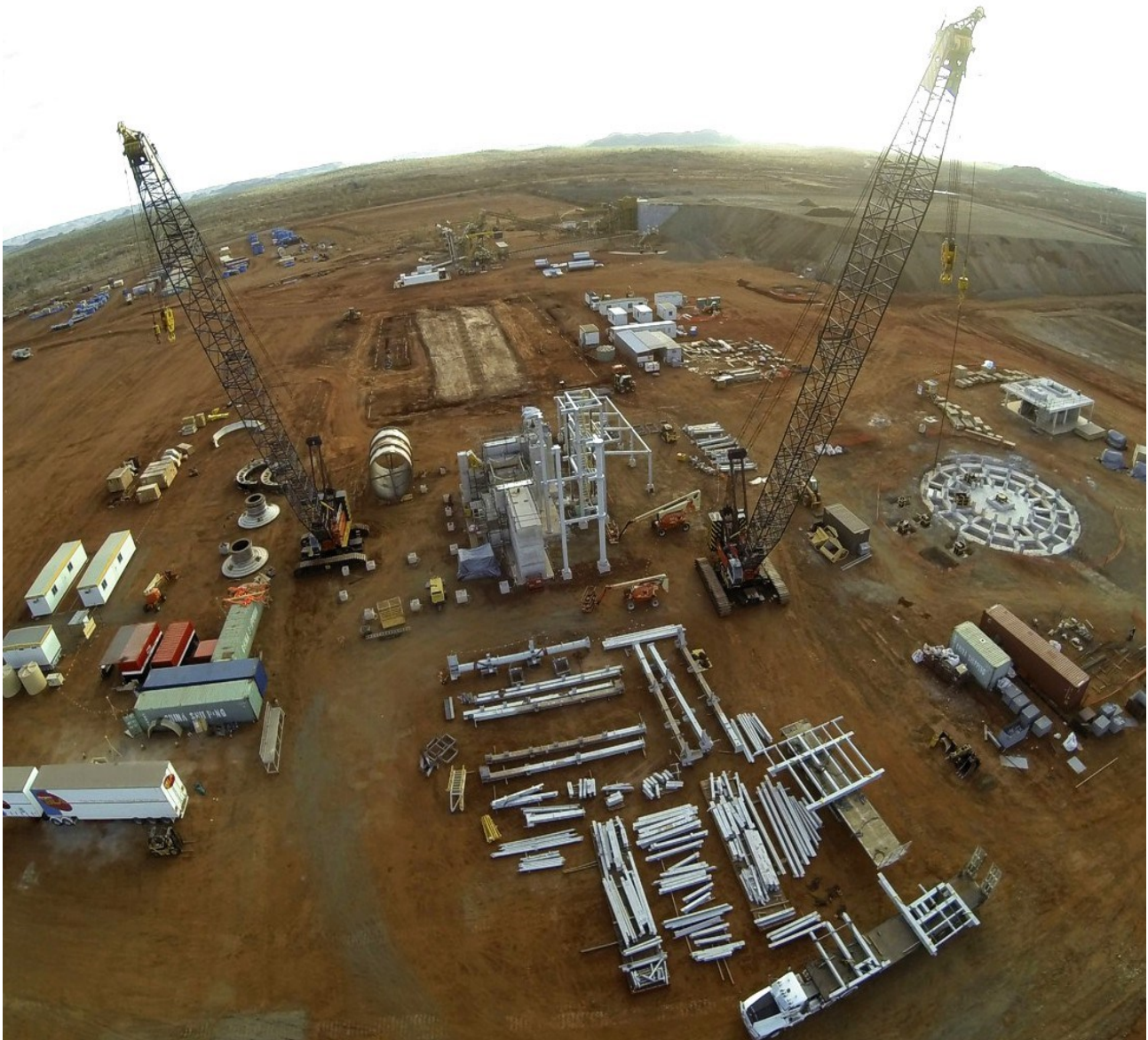
Figure 2: Birds-eye view of the Rocklands Processing Plant, with the Ball Mill structure centre, prior to the lift.
