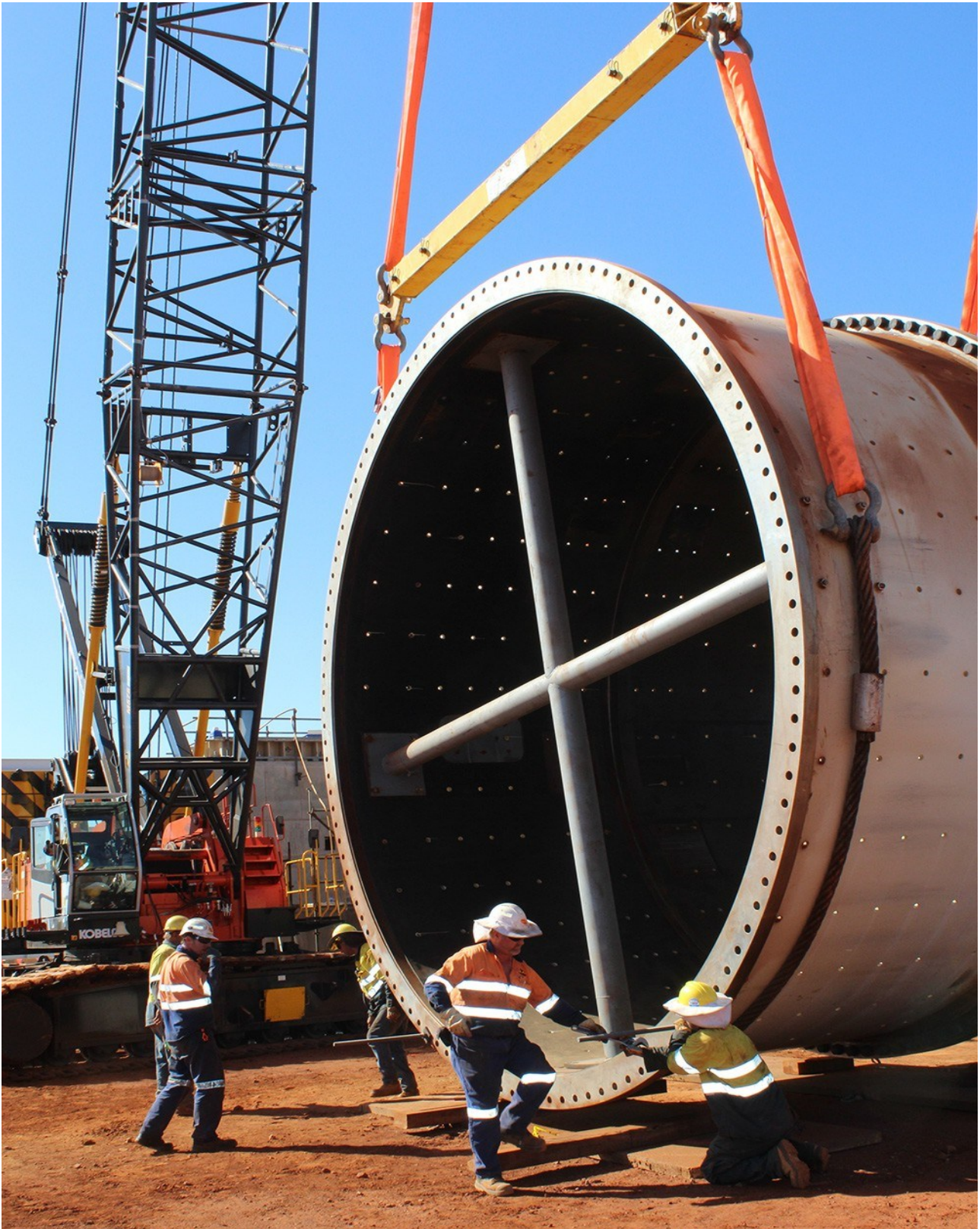
Figure 3: Primary Ball Mill - concrete housing and foundations (left behind crane) and drum segments in the foreground dwarf the lifting crew as they prepare for the lift.
