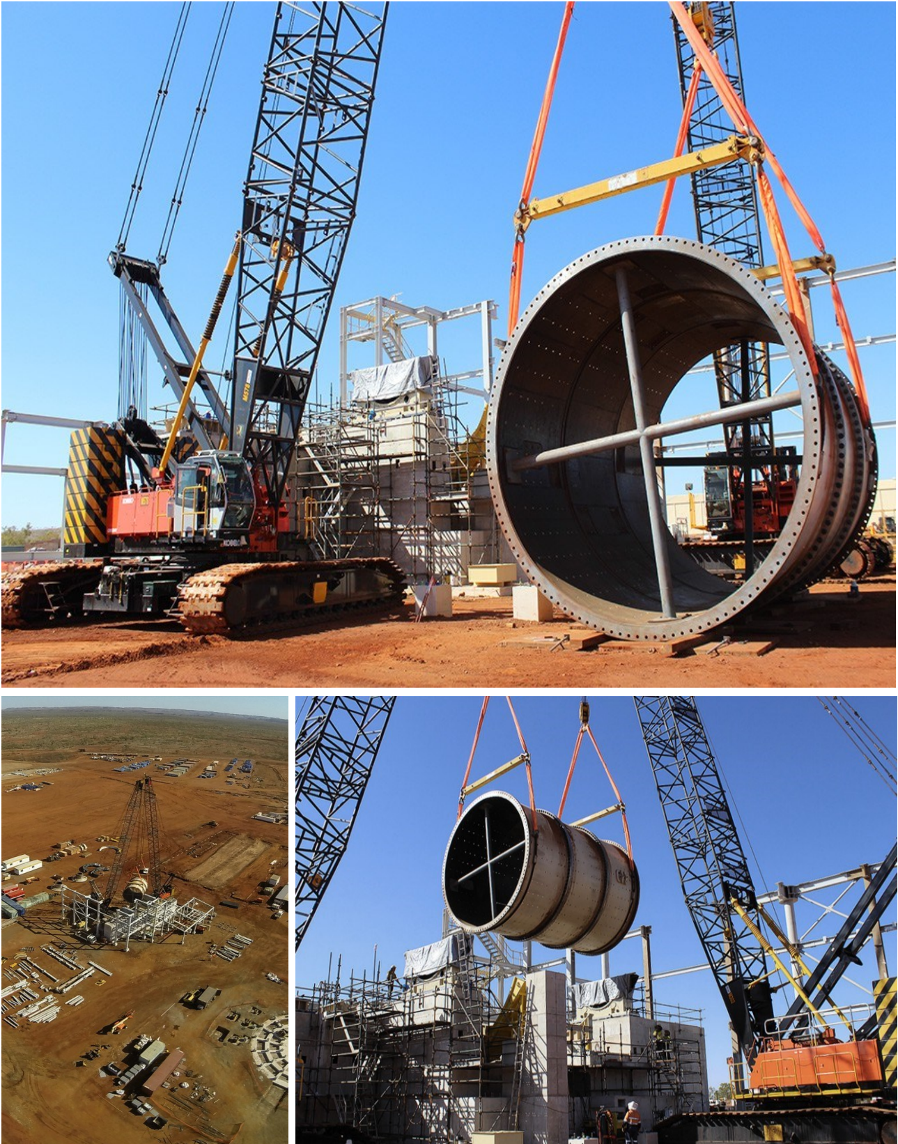
Figure 4: Various views of the Ball Mill lift in action.
