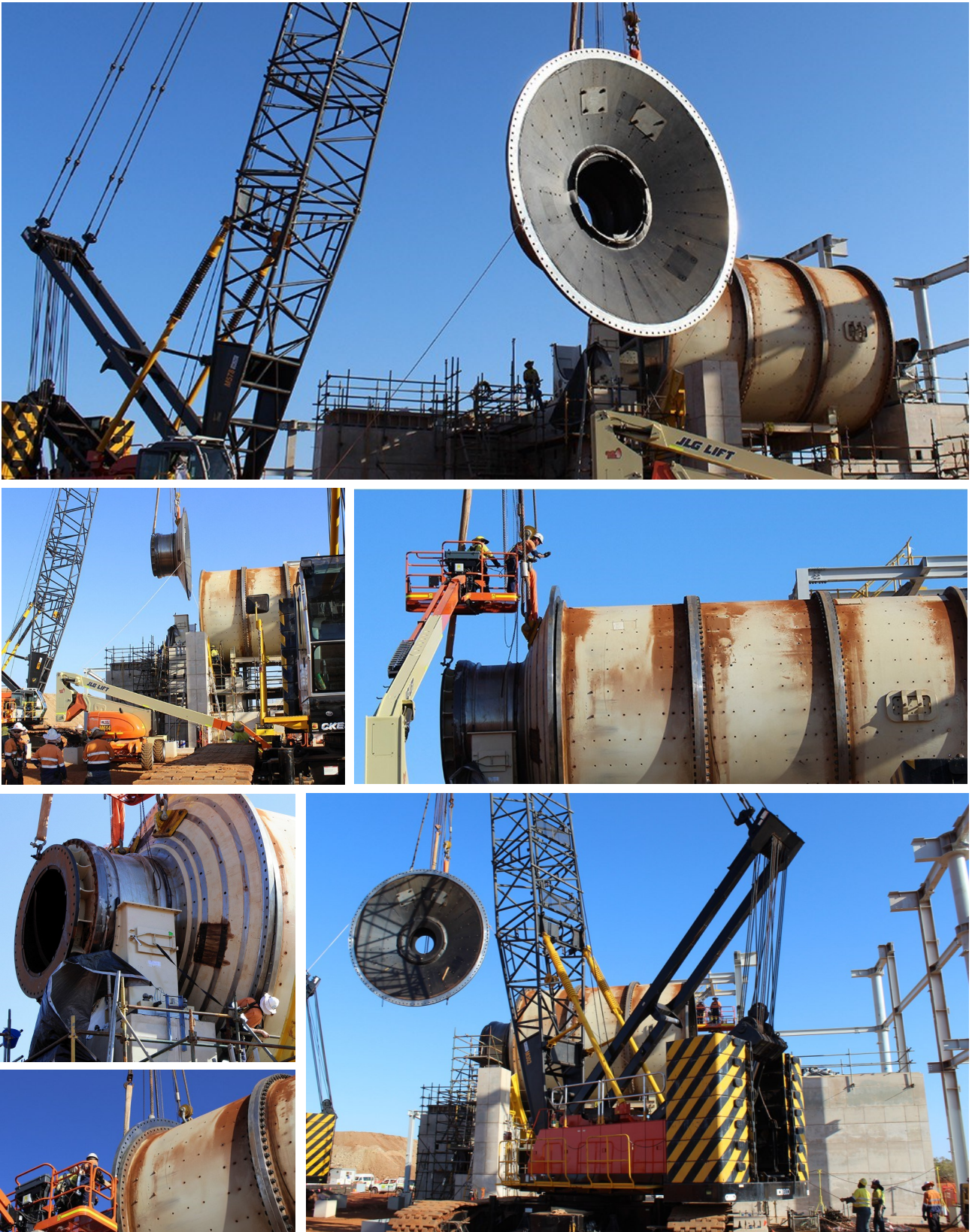
Figure 8: The Ball Mill ends are lifted into place
