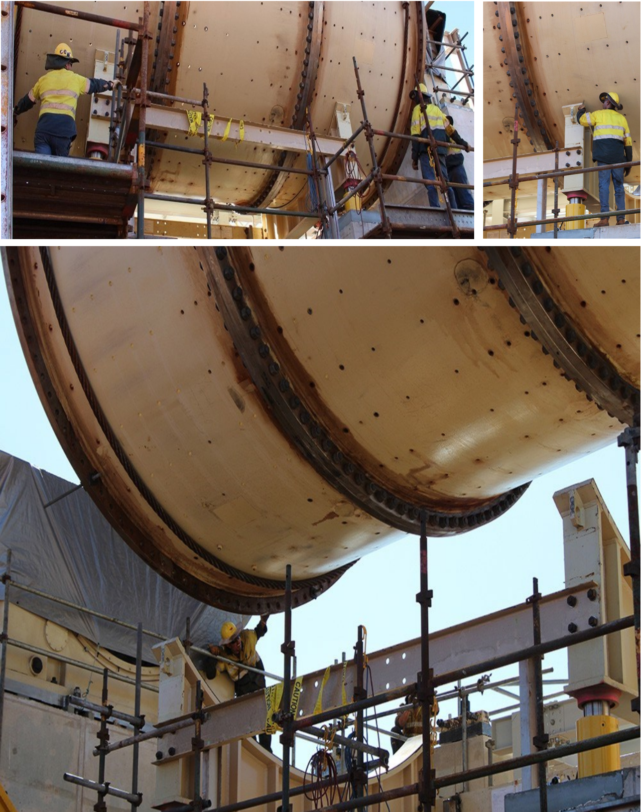
Figure 7: The giant drum is carefully positioned into place prior to the ends being installed.
