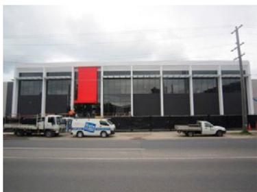
The Property comprises a Data Centre that was completed in August 2012 (although minimal items were still being finalised as at the date of inspection). The landlord owned items include the building "shell and core" (base building) The Data Centre is advisedly targeting a "Tier 3" rating.
