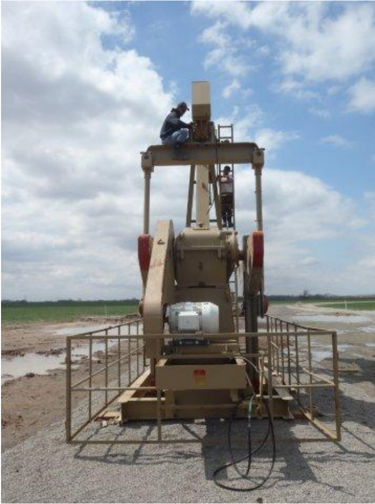
Figure 1 Pump Jack Installation on new well
