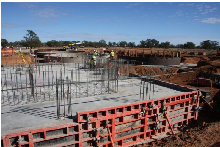
Concrete footings for central plant systems
