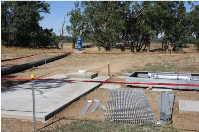
Water production bore and switch footings
