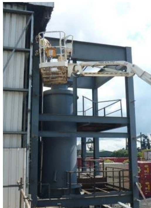
Installation of cleats on the refurbished process tower. The afterburner for the evaporation section has been installed
