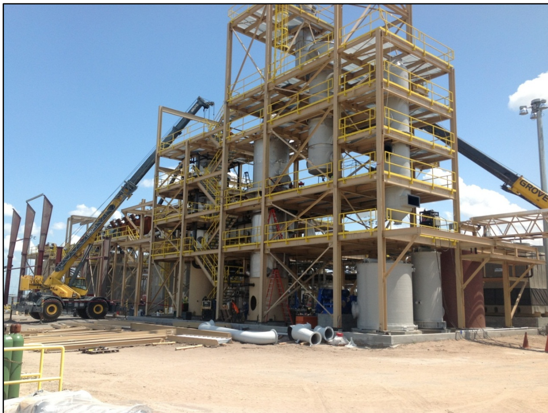
Figure 5: JDCP Demonstration Plant under construction, hydrator in which the SPA will be produced in the foreground – April 2013
