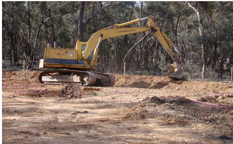
Figure 6. Example of an excavator removing subsoil to create a bund wall around the open pit (Black Reef Mine)
