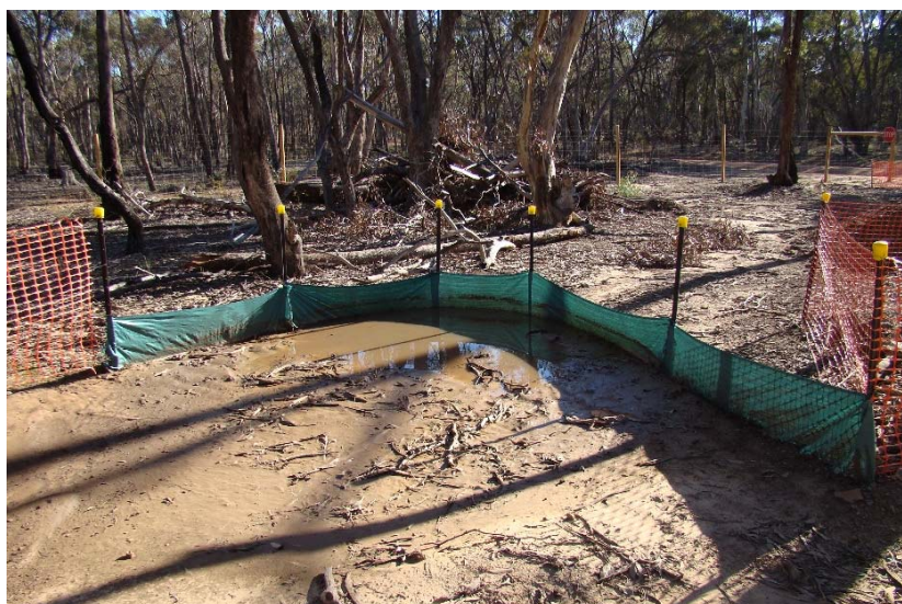
Figure 7. Example of silt mesh preventing erosion, unusable timber stockpiled, & perimeter fence (Black Reef Mine)
