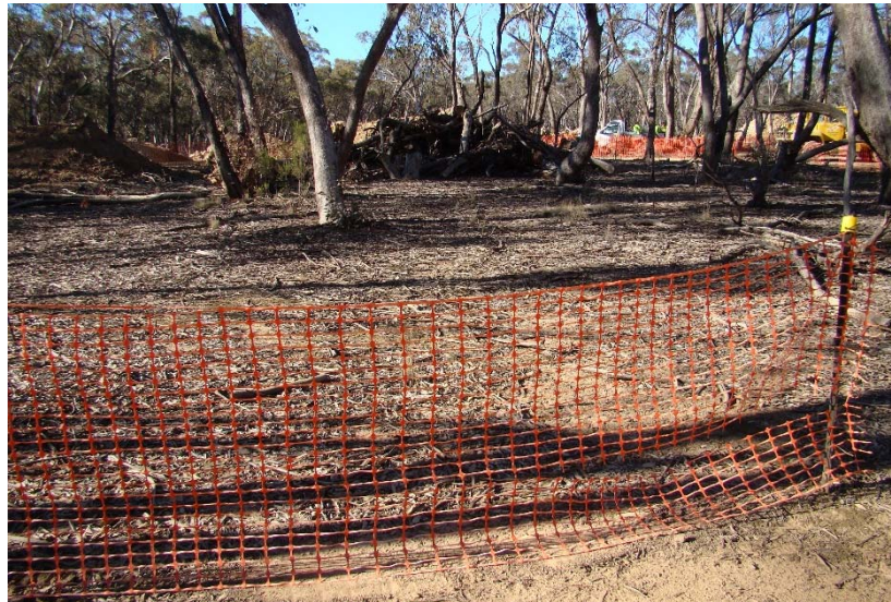
Figure 5. Example of barrier mesh protecting vegetation with unusable timber stockpiled (Black Reef Mine)
