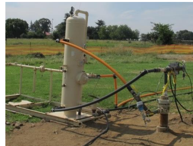
Well head and separator KA-03
