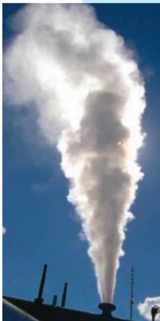
Successful productivity and injectivity testing of the Habanero 4 well. Geodynamics recorded one of the highest reservoir productivity results globally for an EGS well with a flow rate of 39 kilograms per second.
