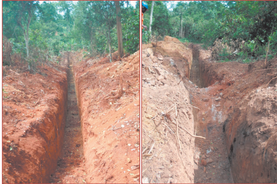
Figure 13. Trenching - 5m Wide Quartz Veining Exposed in Trench at 736800mN on Right
