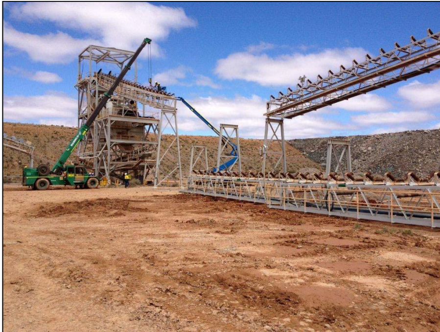
Deconstruction of company owned milling infrastructure located 330km from Murchison
