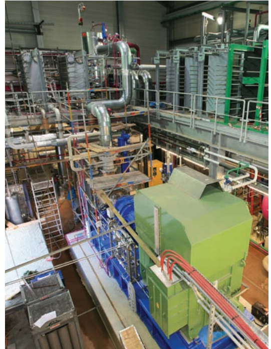
Internal view of Geothermie Unterhaching 3.4 MWe Kalina Cycle® geothermal power plant
