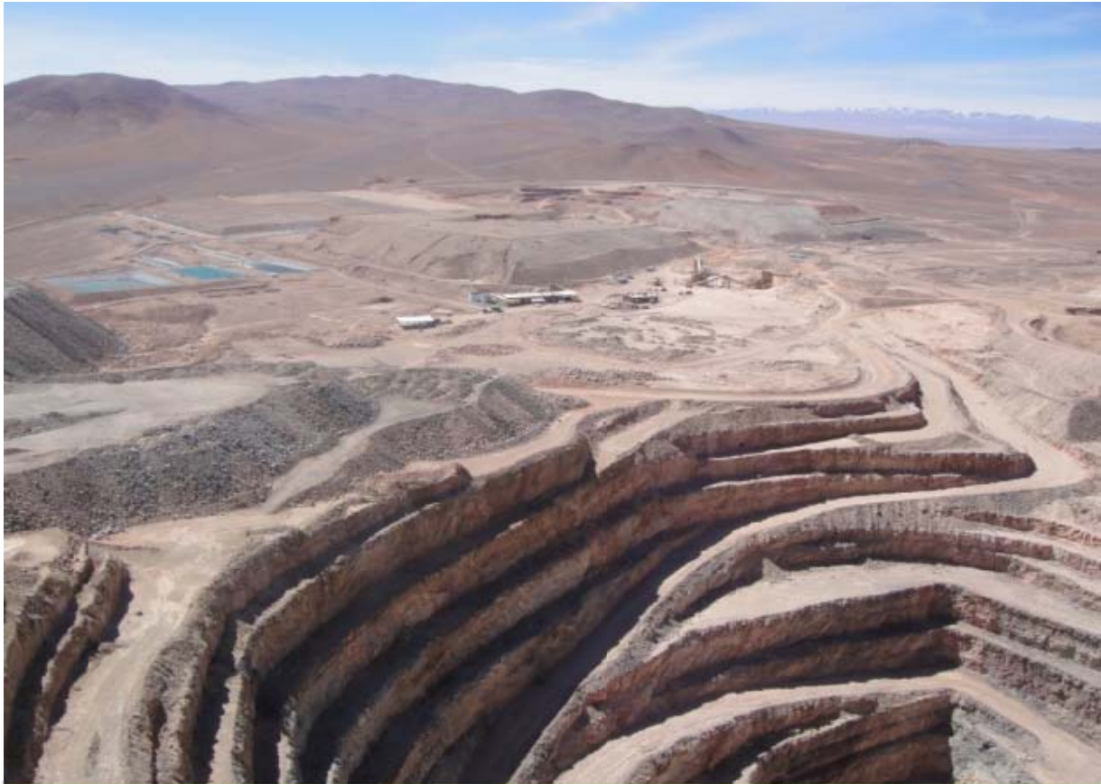
Panoramic view taken from “Cerro Estrella” of the Dumbo Pit and behind it the processing plant, Heaps 1, 2 and 3 and the pregnant solution ponds
