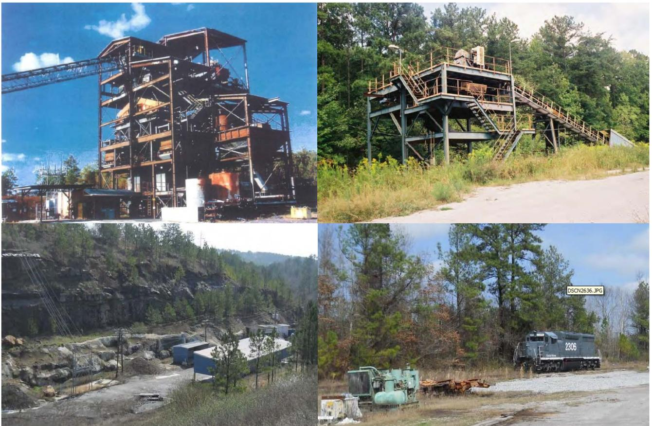
Figure 5: Sample of infrastructure owned by Kodiak; top left - 300tph wash plant, top right - the rail load out facility, bottom left - mine portal and mains power, bottom right – rail spur and locomotive.
