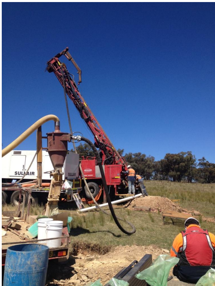
Figure 7 RC drilling at Grenfell in Progress
