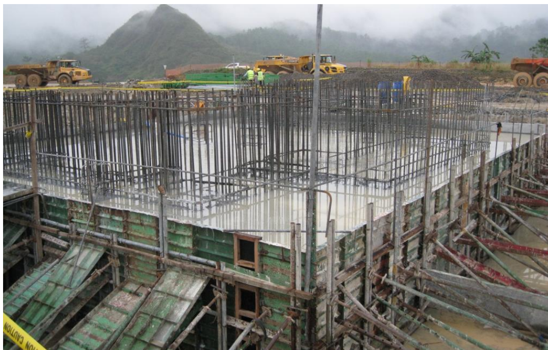
Figure 1: Completed concrete pour for ball mill base
