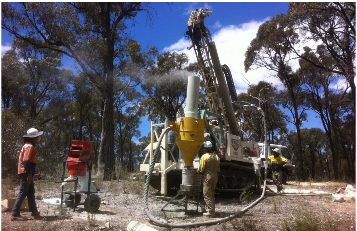
Reverse circulation drilling at Specimen Reef (December 2011)
