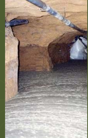
Concrete Pumping for Mine Void Backfilling
