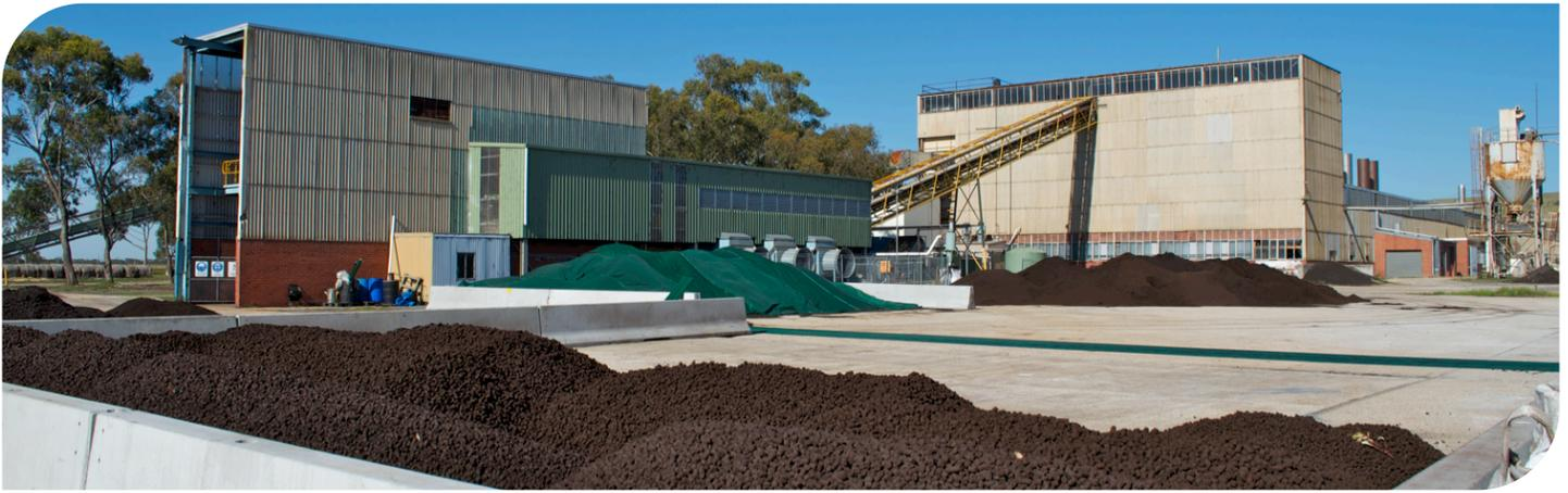
The Coldry Pilot Plant, located near Bacchus Marsh, Victoria has undergone significant activity as part of the Design for Tender program being conducted by Arup. The foreground shows Coldry pellets while raw Loy Yang coal sits in the background waiting to be processed.
