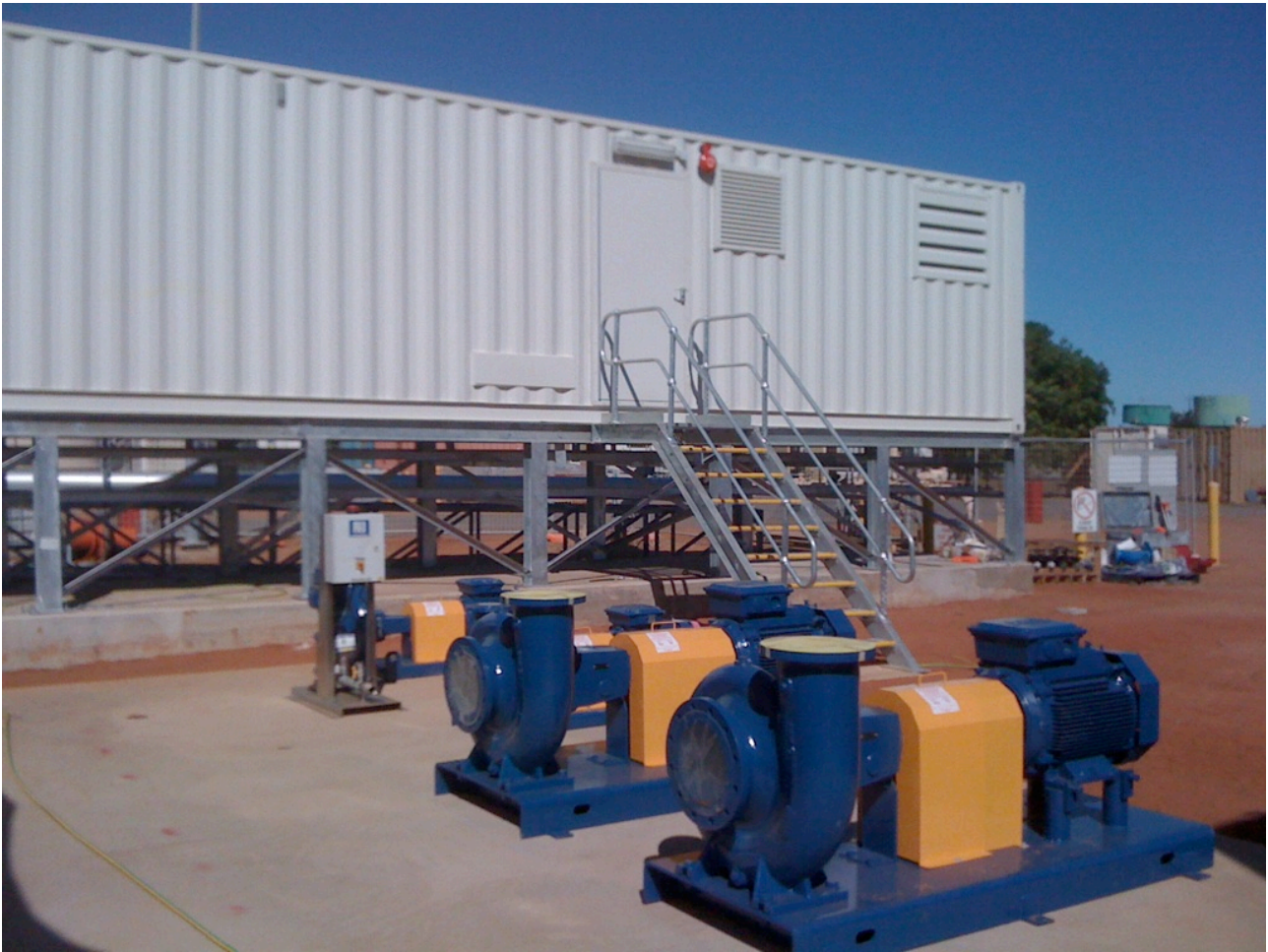
Figure 2 - The switch room installed on its bas with the circulation pumps in the foreground
