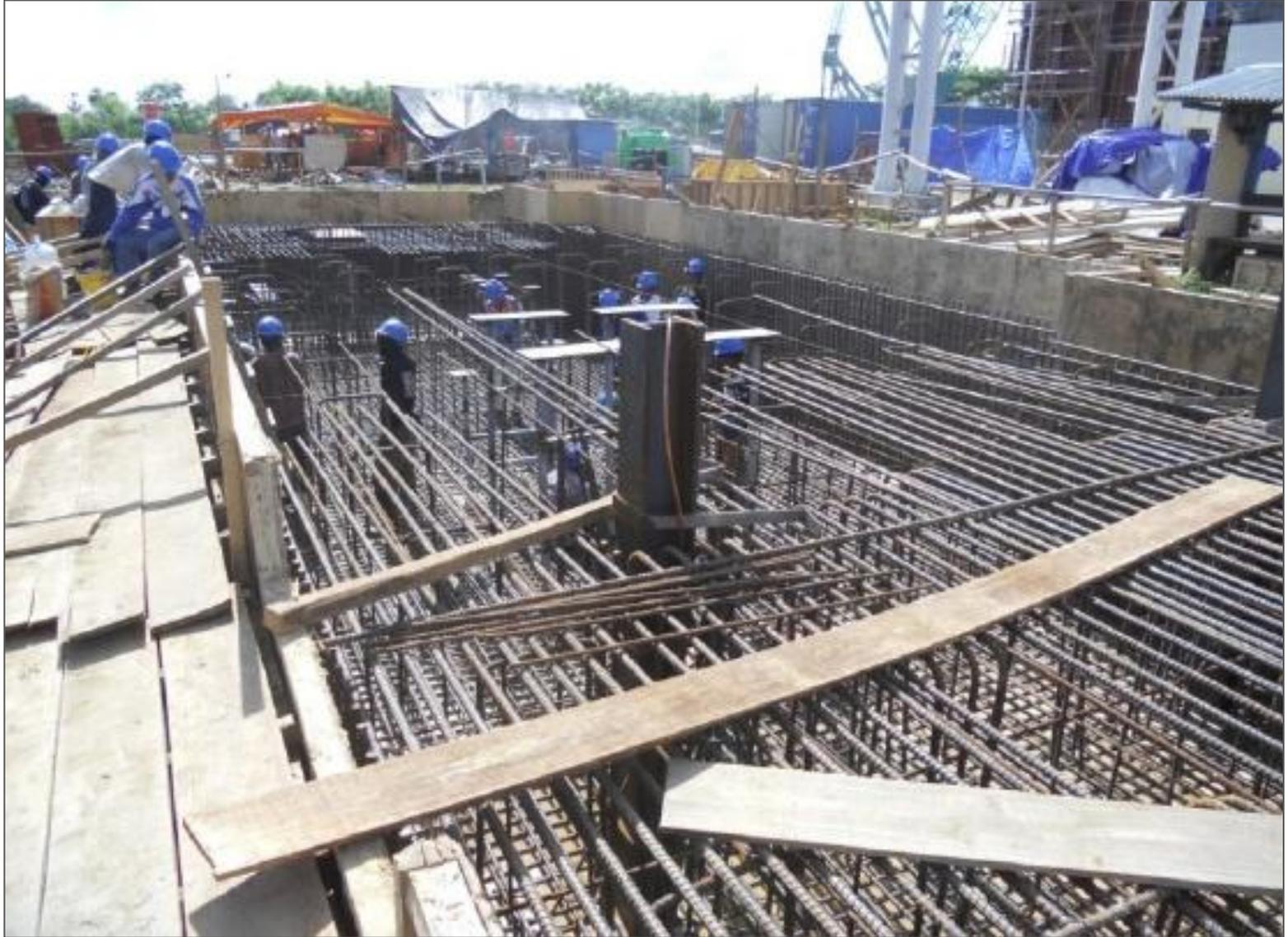
Install for rebar for ST-28 foundation stage-3
