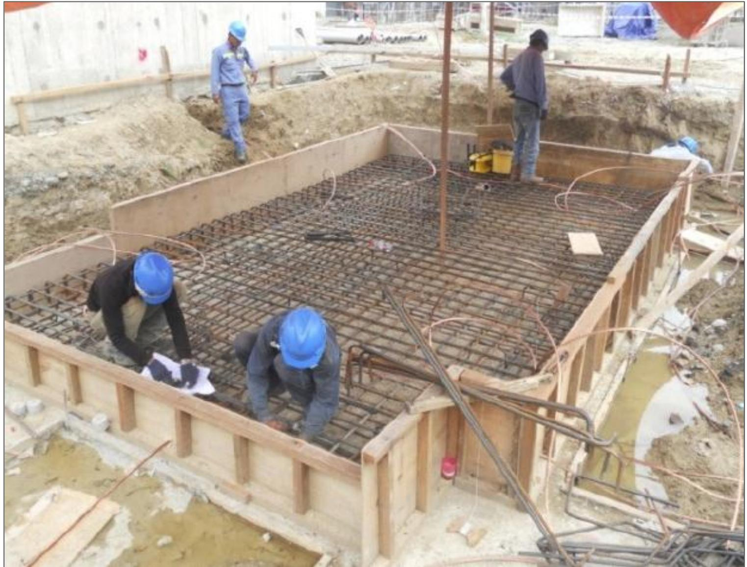
Install rebar for plate foundation of generator circuit breaker
