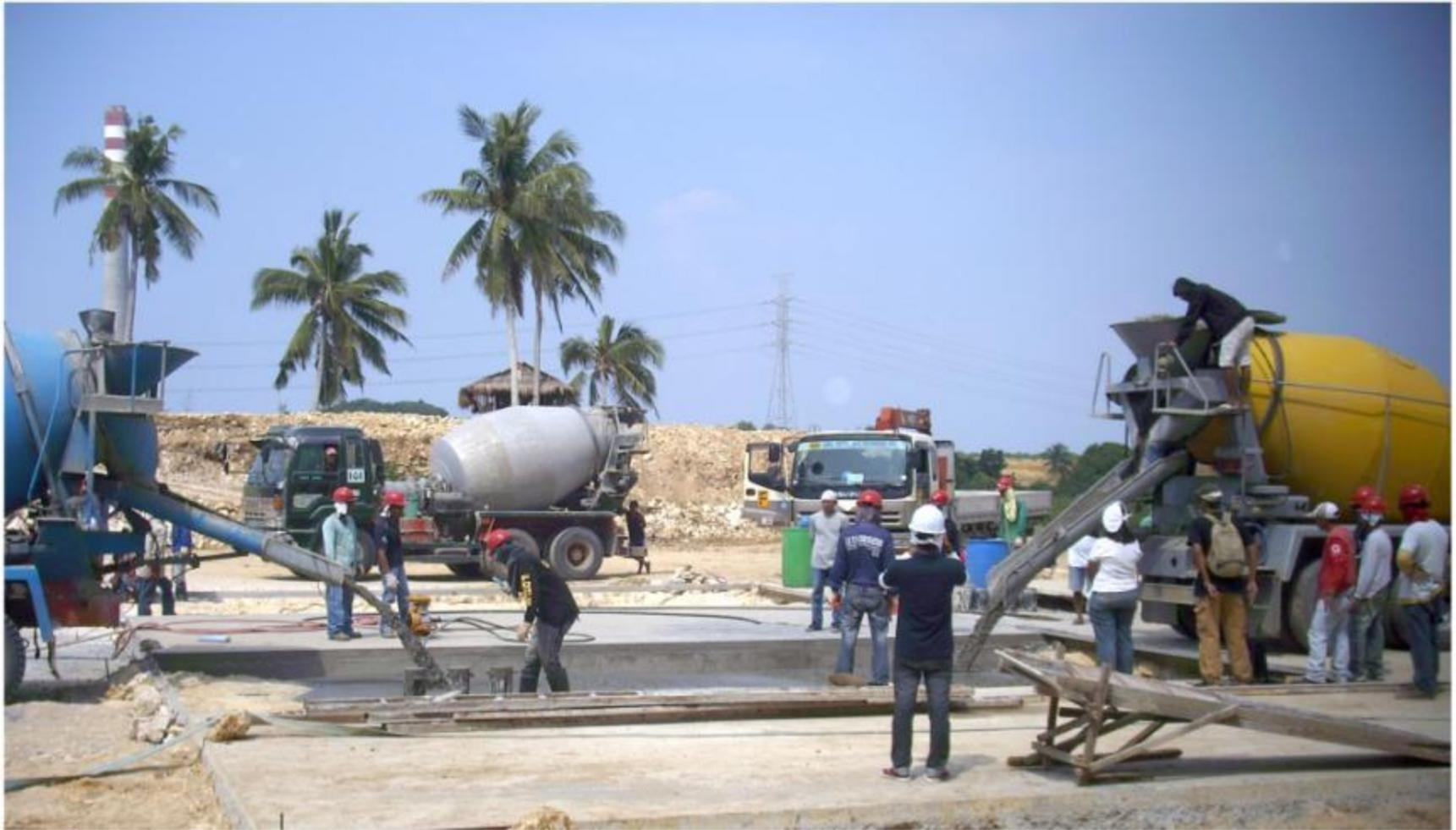
**Pagbilao Pouring Concrete Blinding for The LNG Tank Base Slab.**
