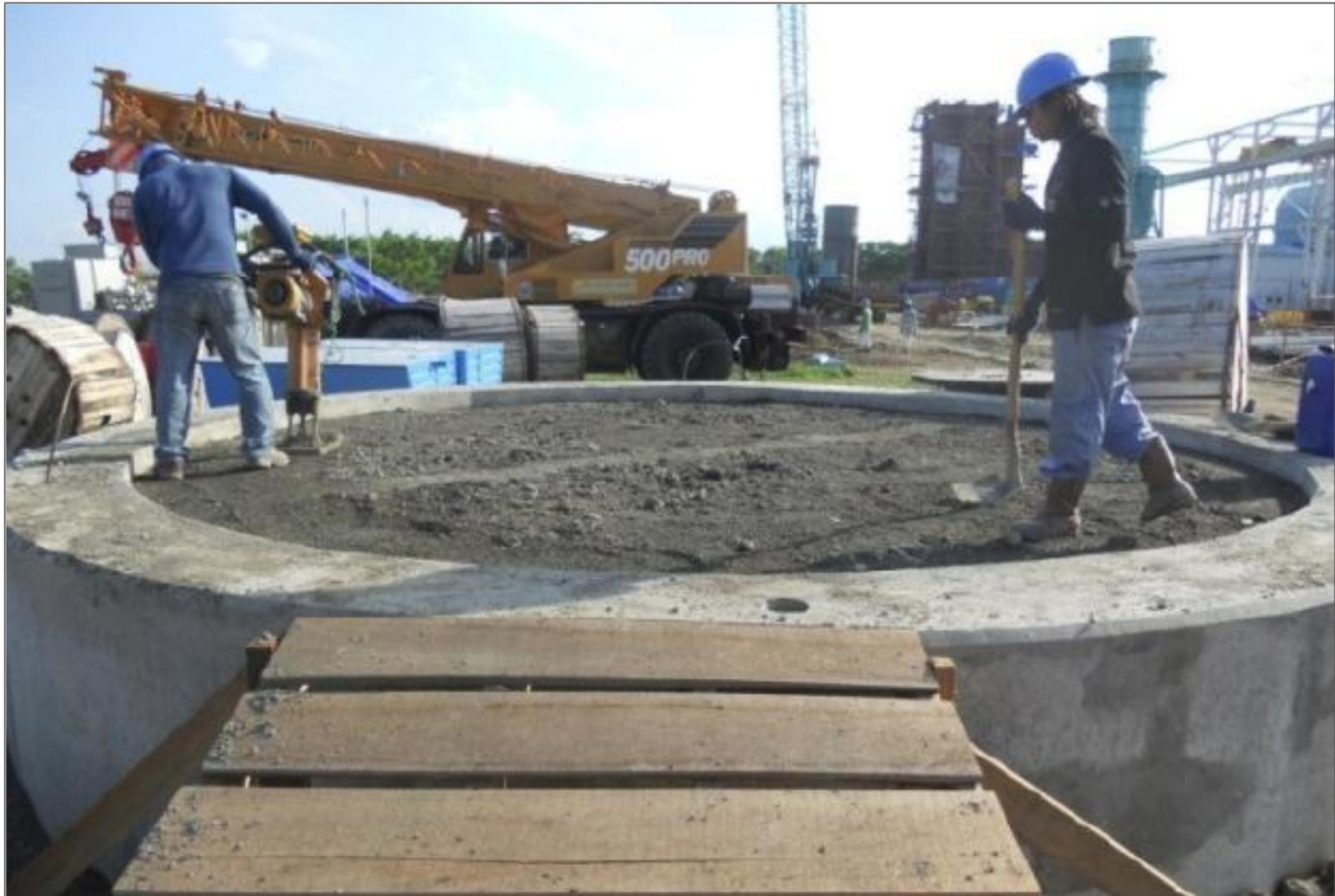
Gravel laying and compact in the Ring foundation of demineralized tank
