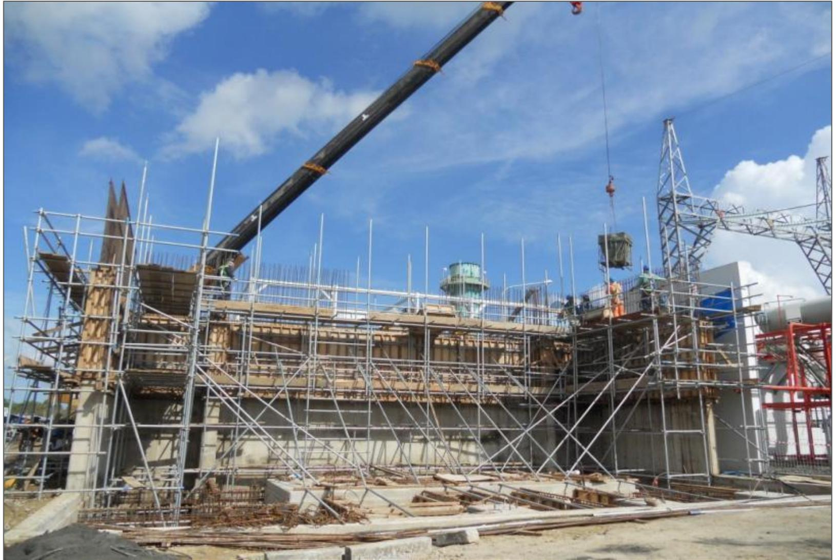
Pouring concrete for blast wall ST-28 main transformer step-2
