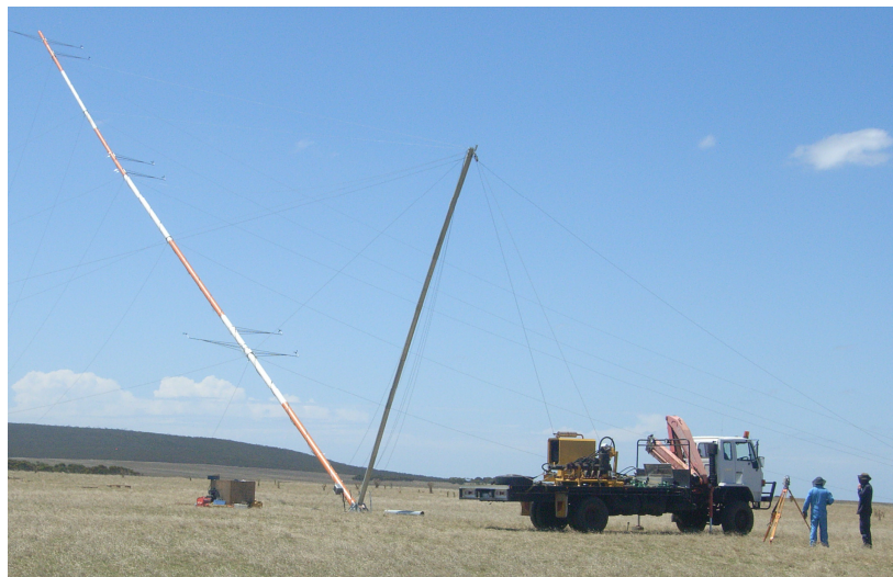
FIG 1- Wind Tower Erection- Trilogy
