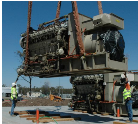
Gas engines being positioned On site
