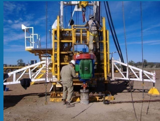
Installing an electric drive head
