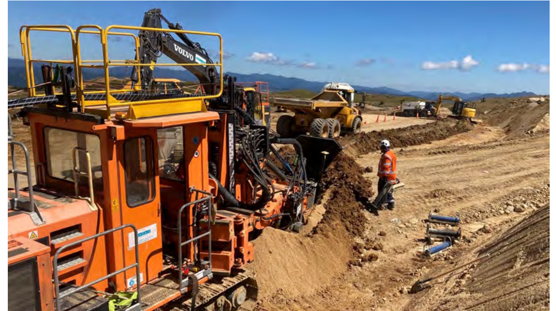
Cable trenching at Meridian's Harapaki wind farm
