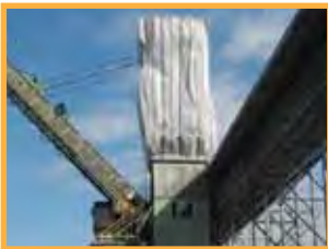
Protective Coatings (Blast & Paint)
