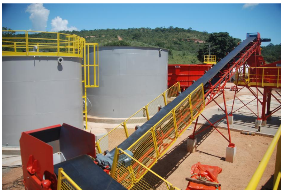
Figure 2. View of process and potable water storage tanks (grey in foreground) and the tailings thickener (red in background)
