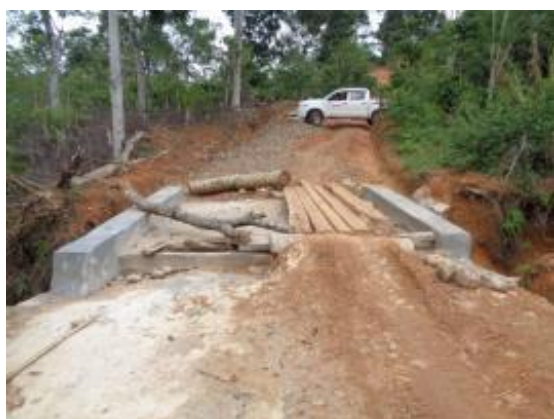
Picture 2: Repair of Petai Kayu bridge
