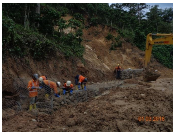
Picture 5: Erosion control in areas affected by landslides
