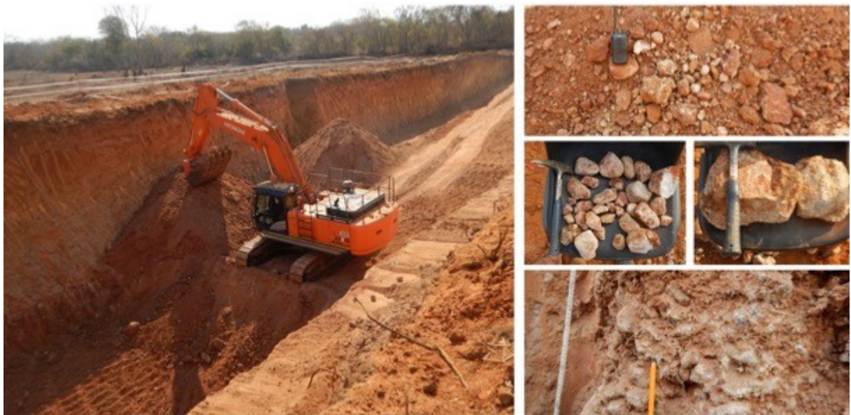
Figure 6. (i.) Excavation of Alpha Pit – depth Dug area up to 9.2m (ii.) Gravel layer in the stock pile (iii.) Gravel clasts of quartzite ranging from 2cm to 8cm in diameter (iv.) Angular quartzite clasts approximately 15 cm in diameter and (v.) Gravel layer (red oxidised material with quartz clasts)
